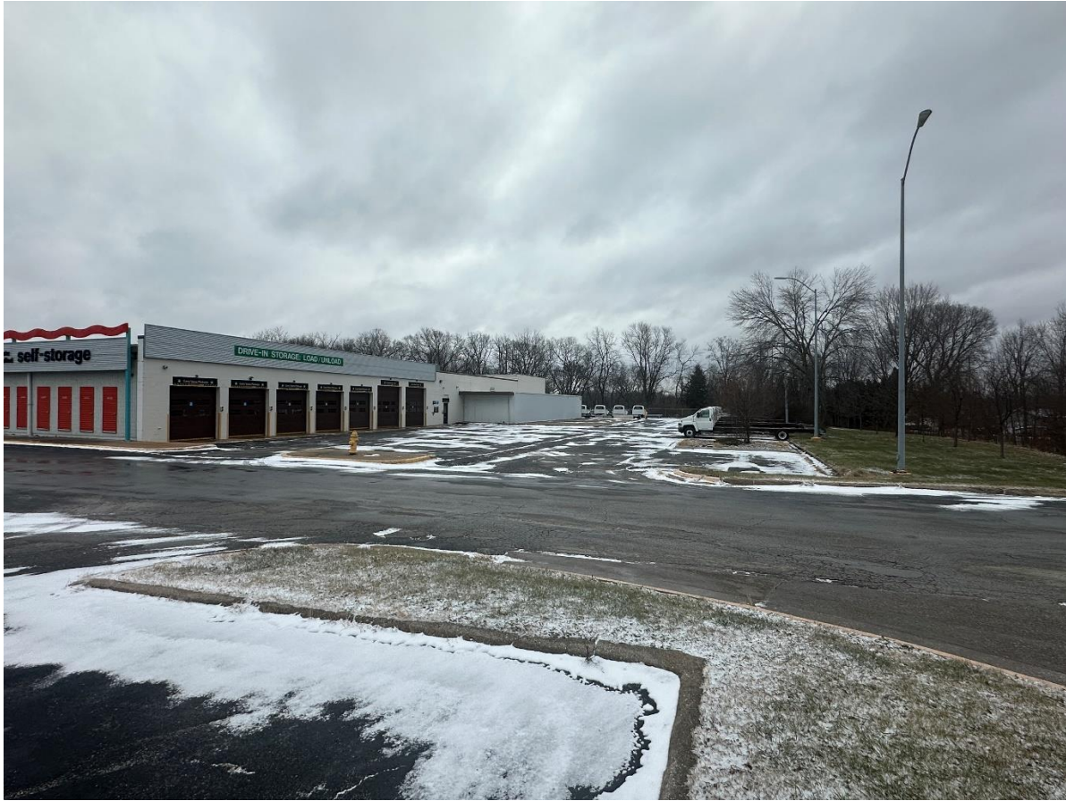
Figure 2: Photo showing area east of the building where the storage units are proposed to be located.
