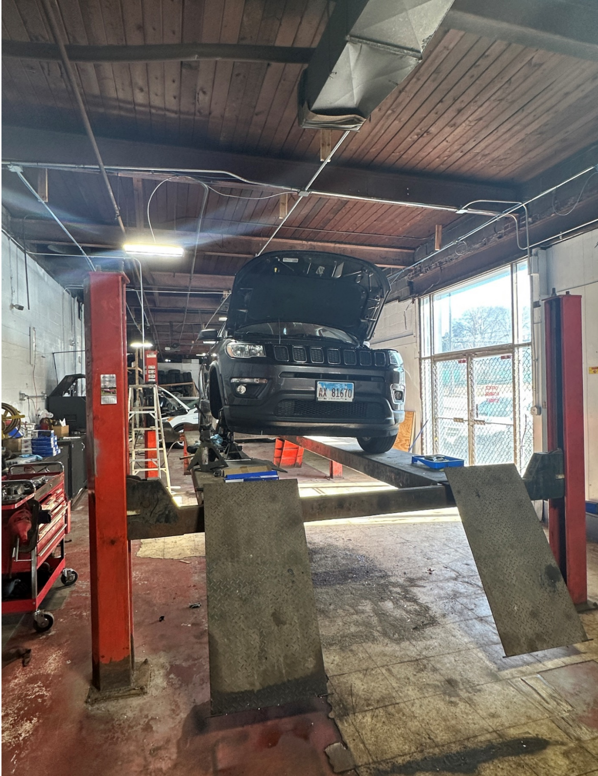
Figure 3: Photo showing the setup in the building
