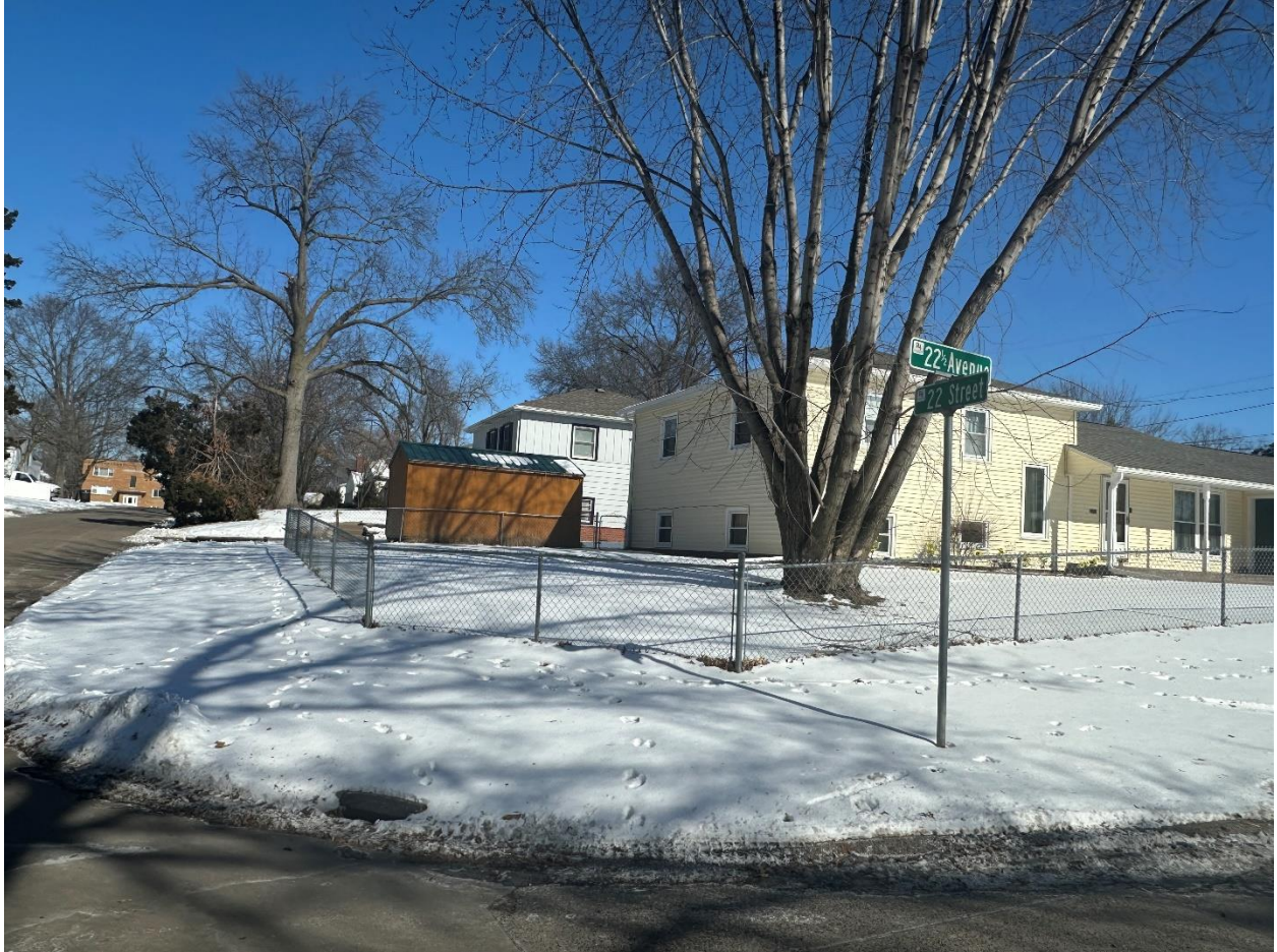
Figure 1: Photo showing shed from along 22 ½ Avenue
