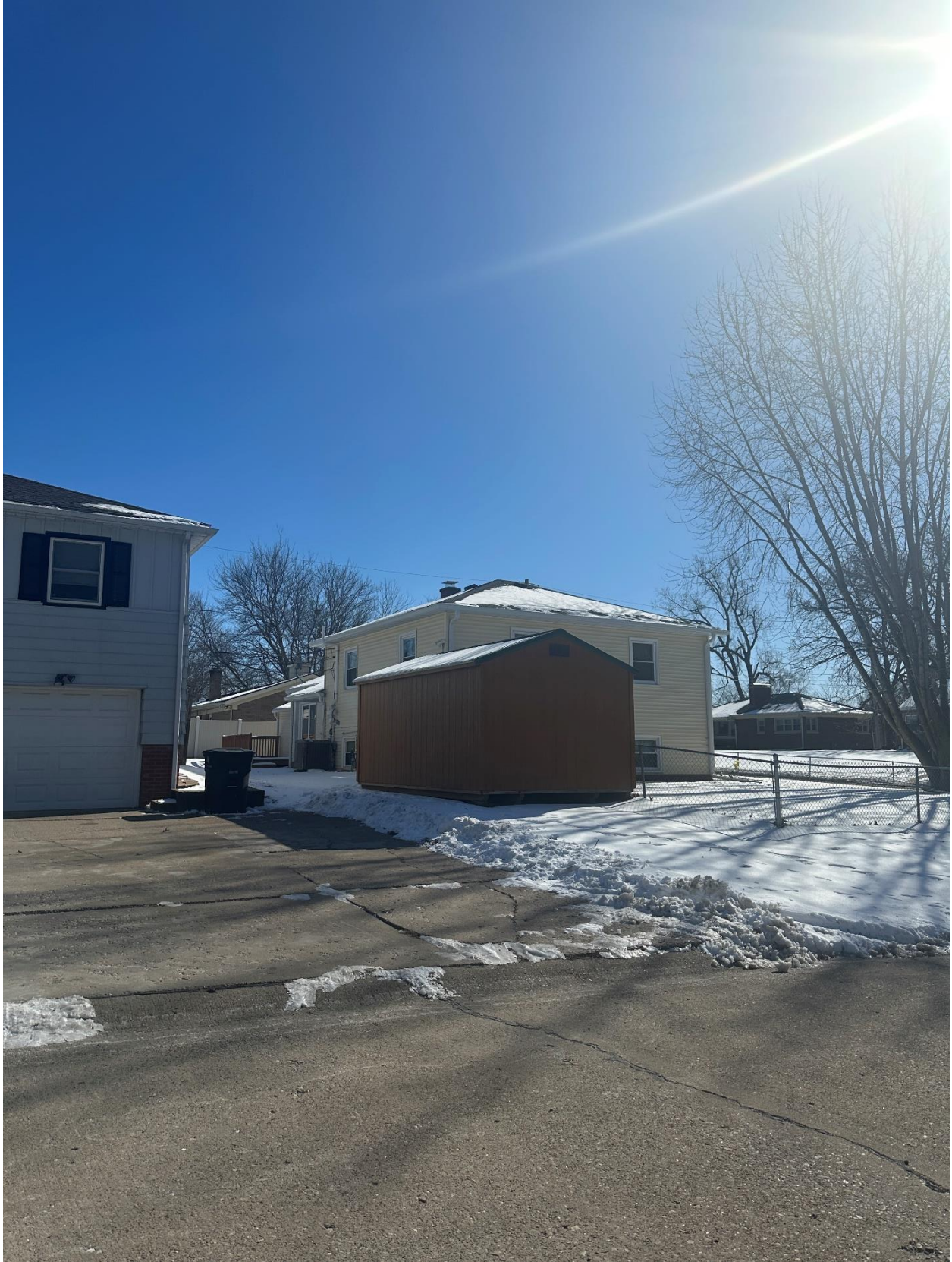
Figure 2: Photo showing shed from along 22 nd Street
