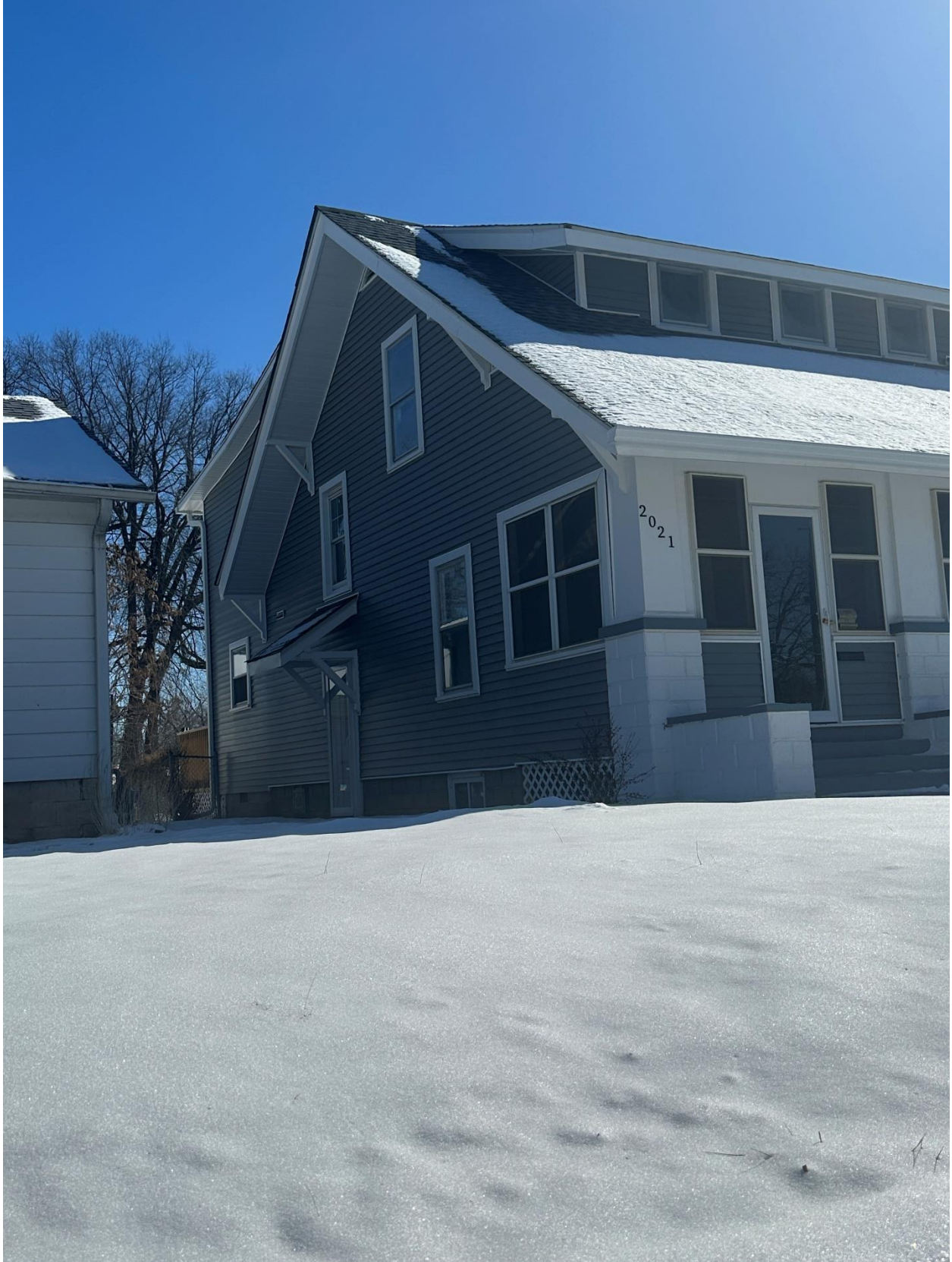
Figure 2: Photo showing the side door which will serve as the entrance for clients
