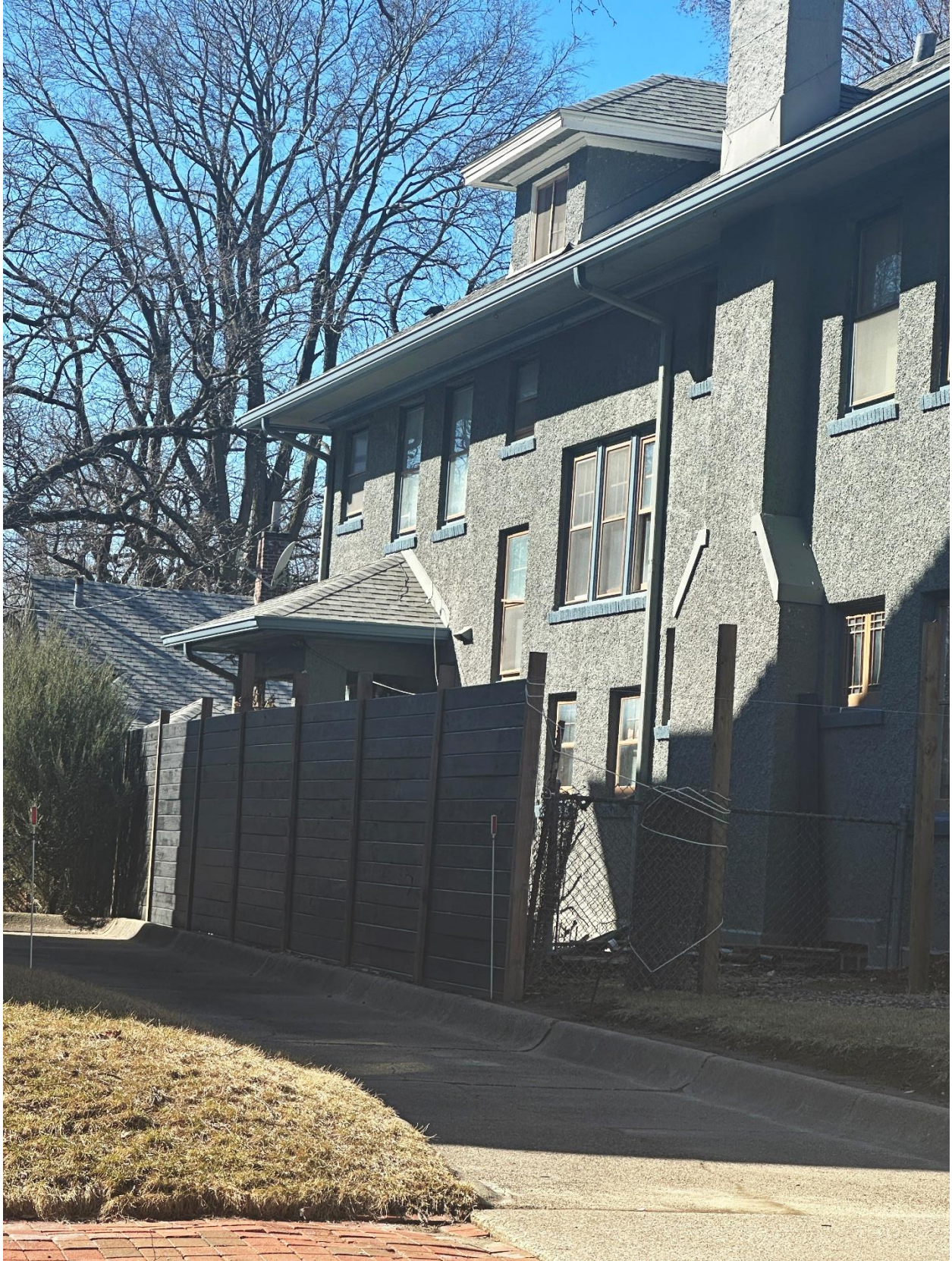
Figure 1: Photo showing the fence from along 22 nd Street
