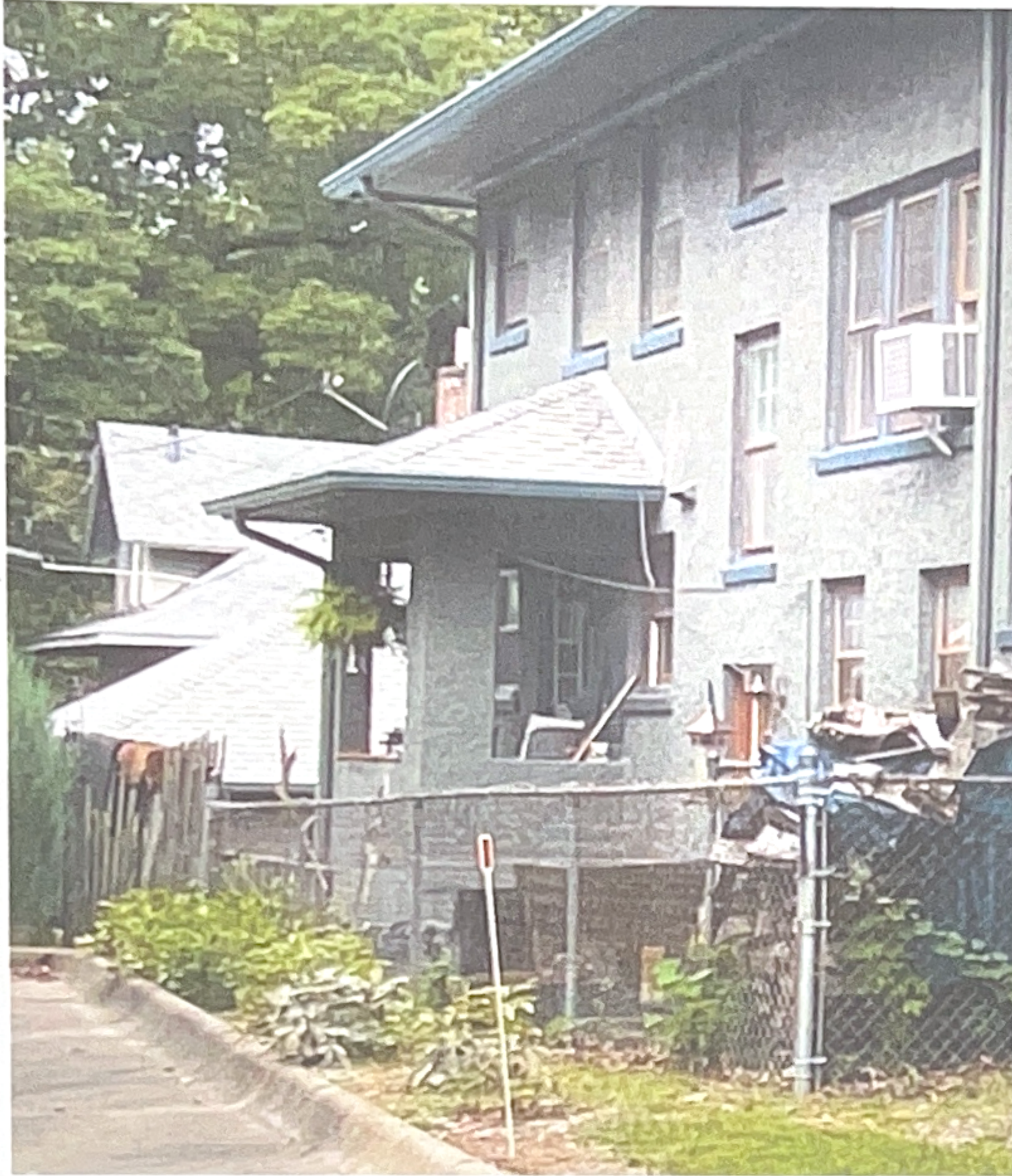
The above photo is of the original fence, partial chain link 4 feet and 6 feet vertical wood.
