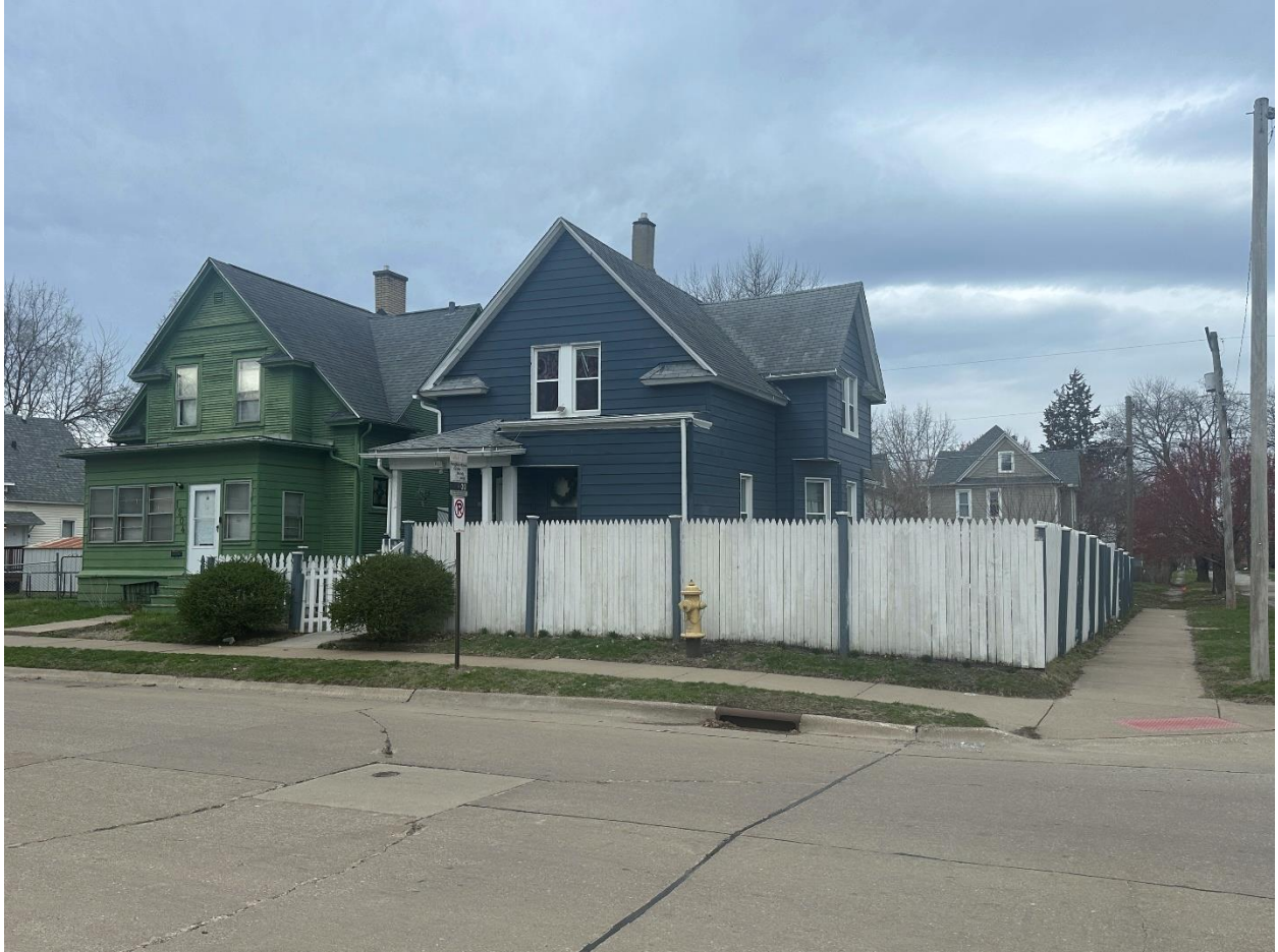
Figure 1: Showing front of house with 6ft fence from along 15 th Street
