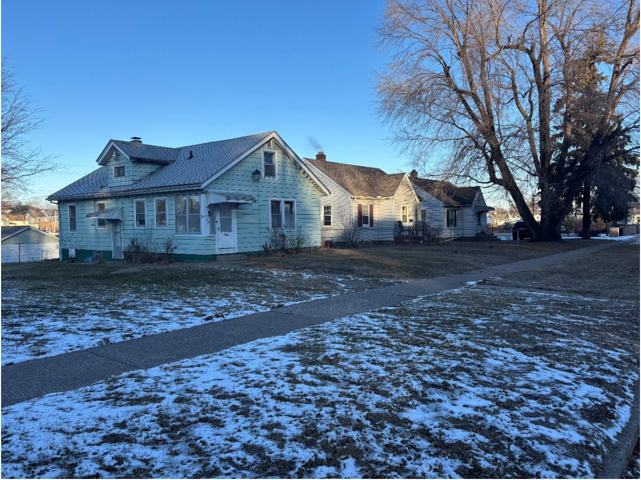
Figure 3: Looking northwest at the subject property.
