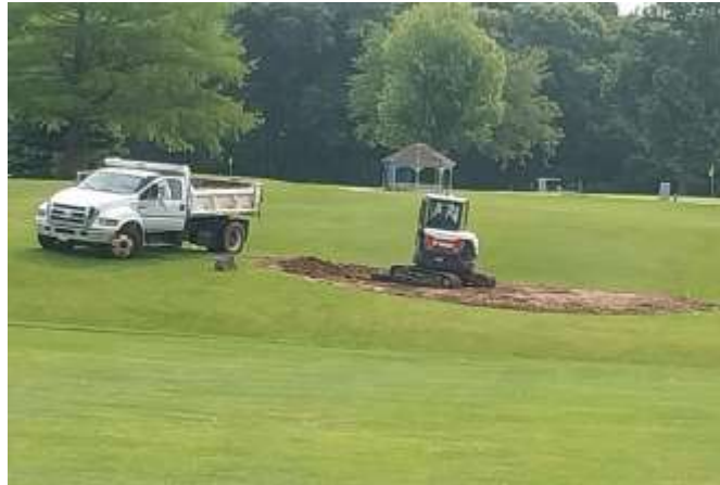
#7 tee box beginning renovation
