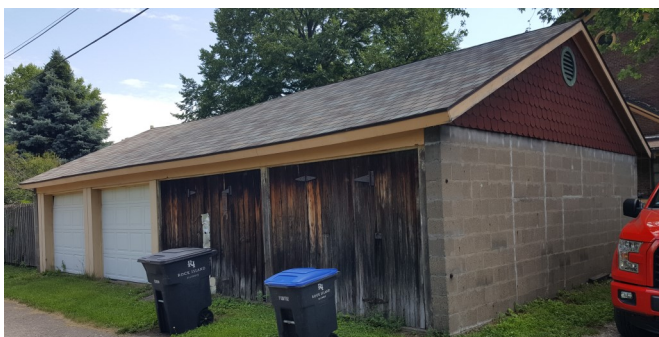
Fig.13. Garage, alley side (left)
