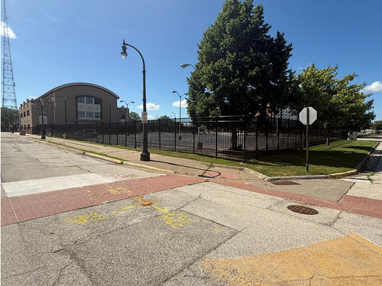
Figure 5: Photo showing installed 8ft fence along 3 rd Avenue
