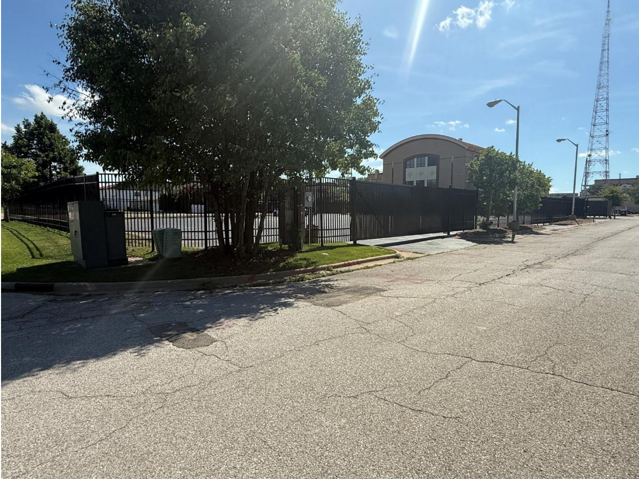
Figure 3: Photo showing installed 8ft tall fence along the alley
