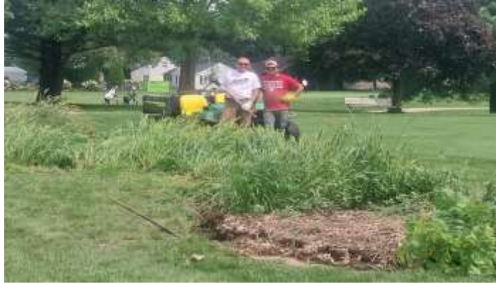
Removing retaining wall blocks behind #2 tee box
