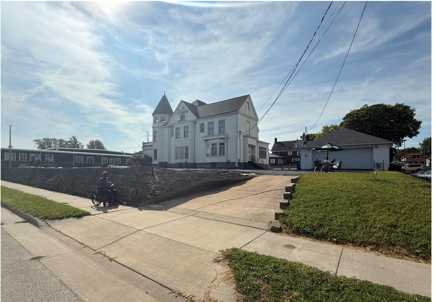
Figure 5: Photo showing property 608 20 th Street (building) from the north-west perspective
