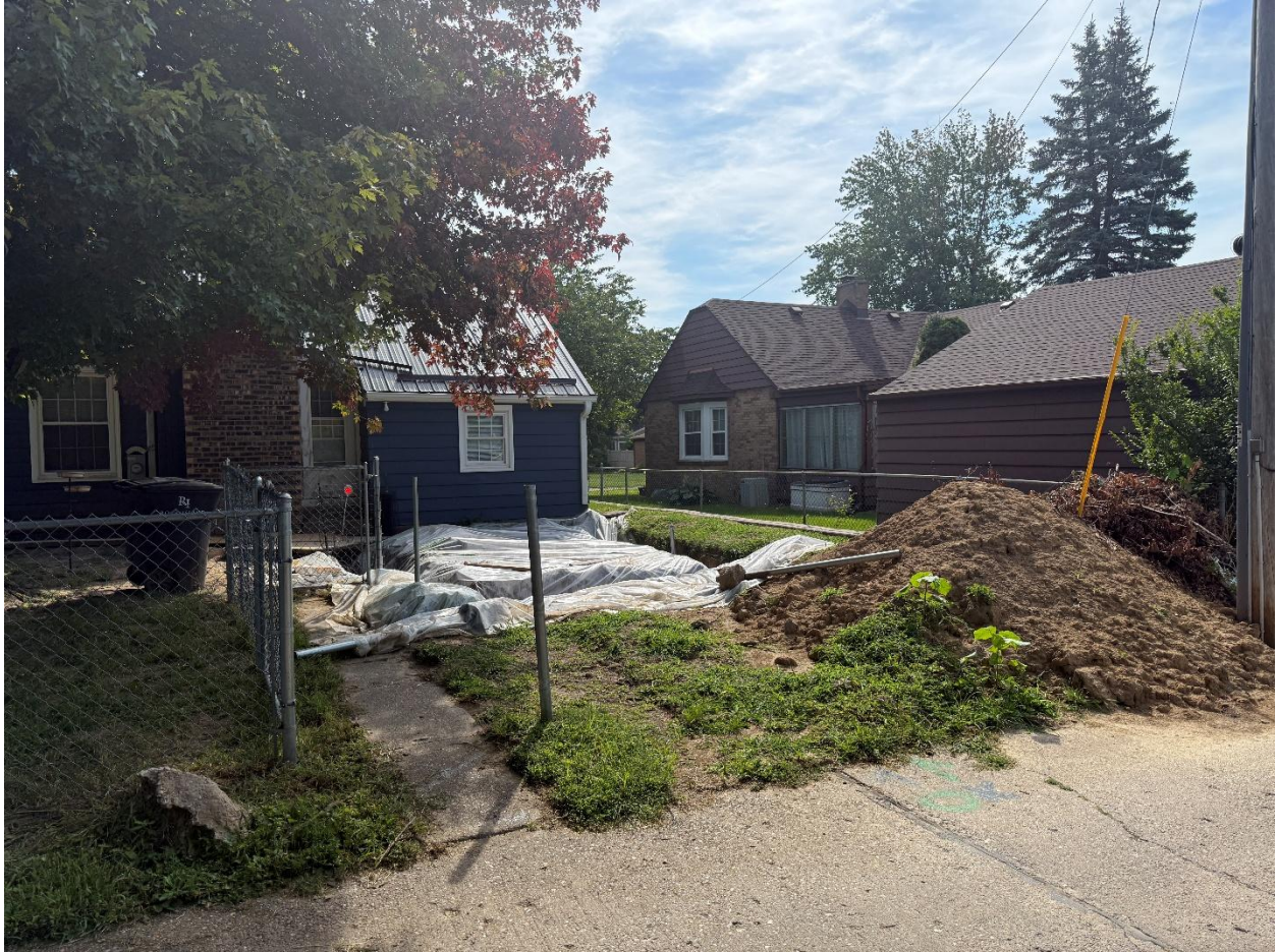
Figure 2: Photo showing area dug out for garage addition
