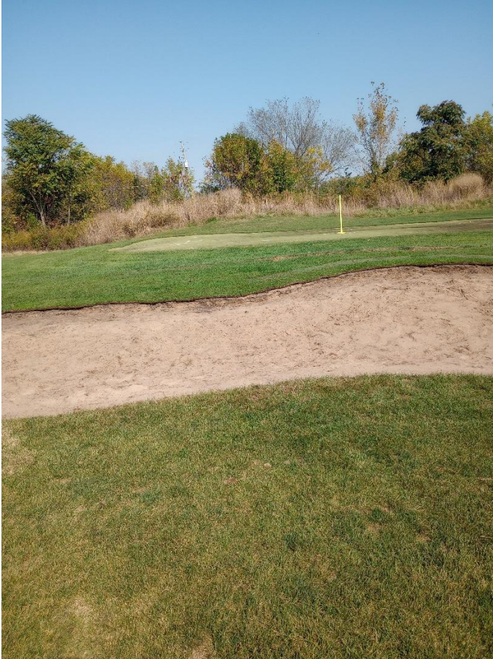
Practice bunker completed.
