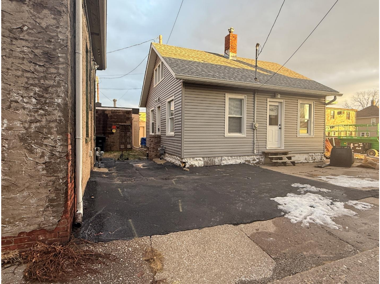
Figure 3: Photo showing distance between the commercial and residential building
