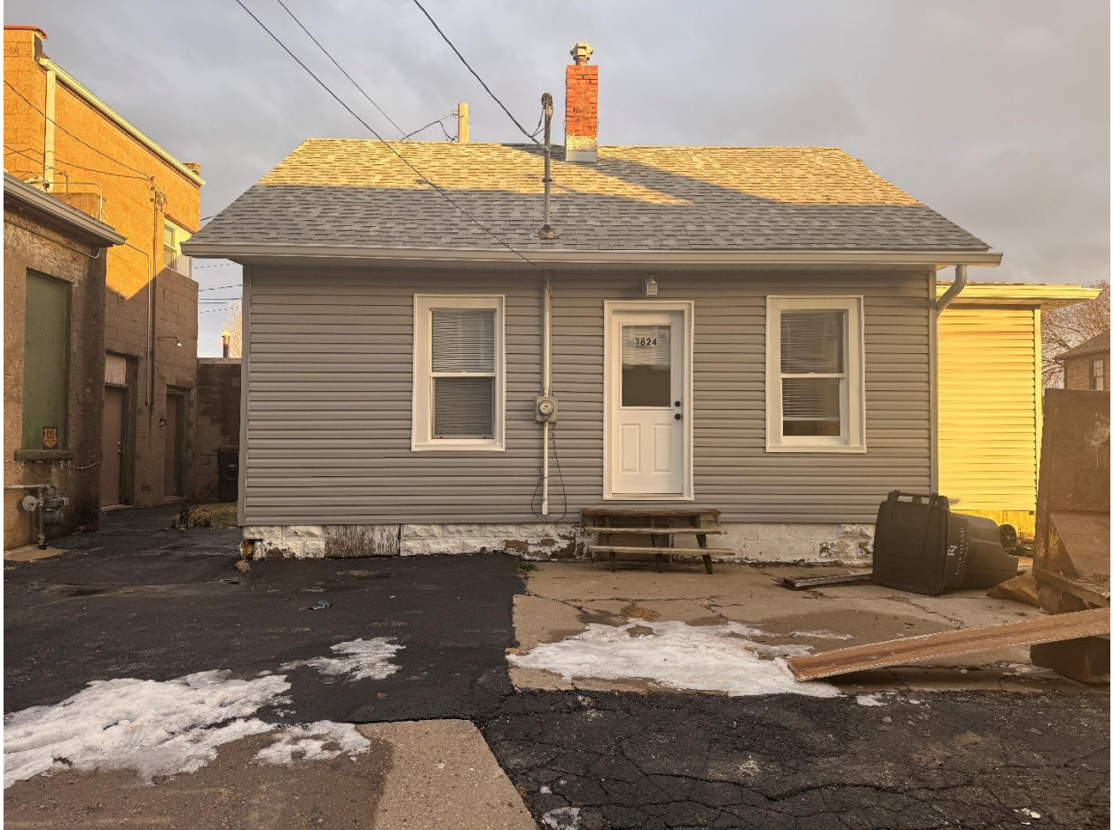
Figure 2: Photo showing residential structure on proposed south lot from the alley
