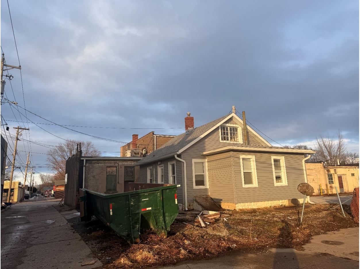
Figure 4: Photo showing properties from the alley
