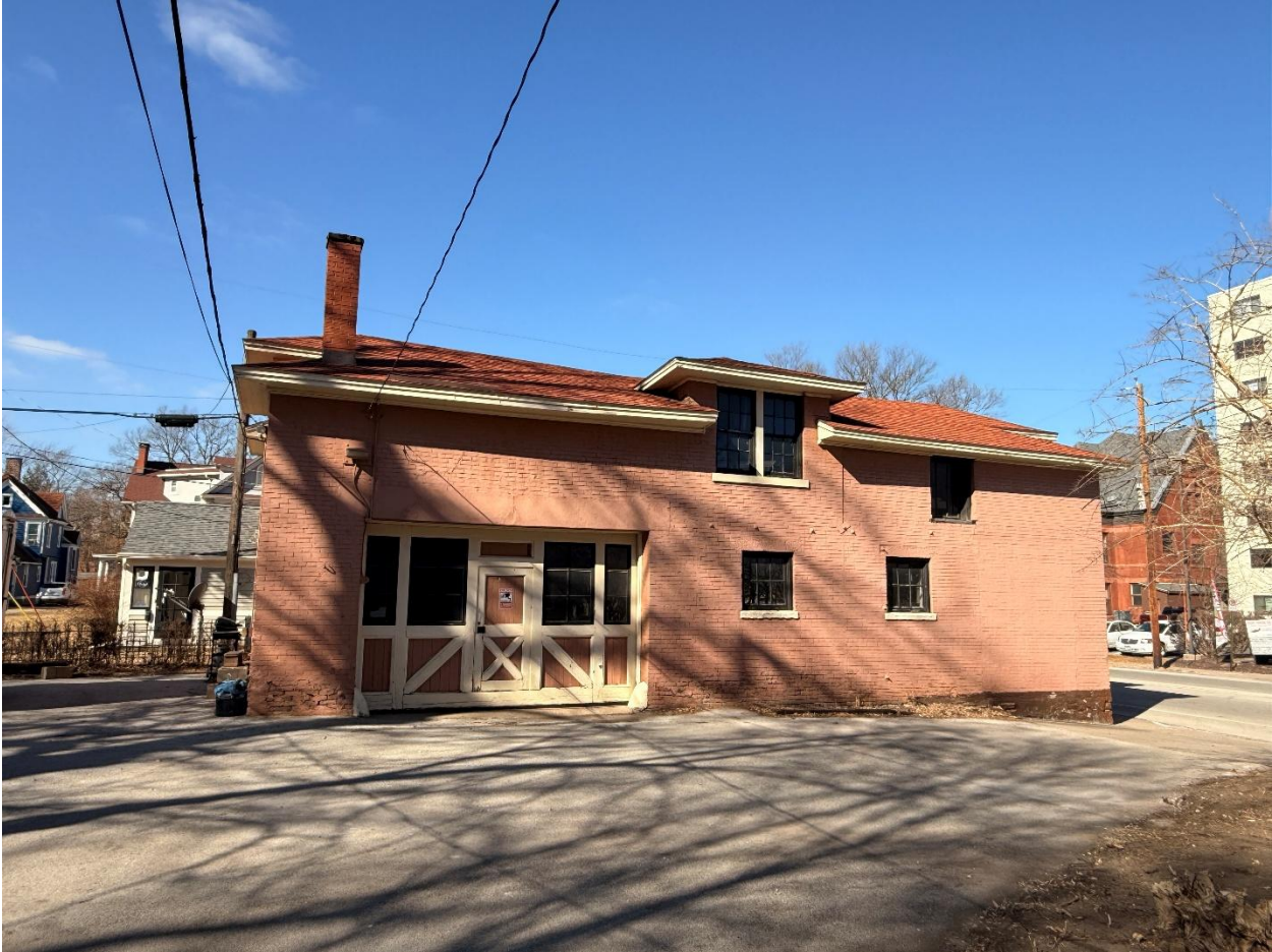
Figure 4: Photo showing parking garage to be used as parking space
