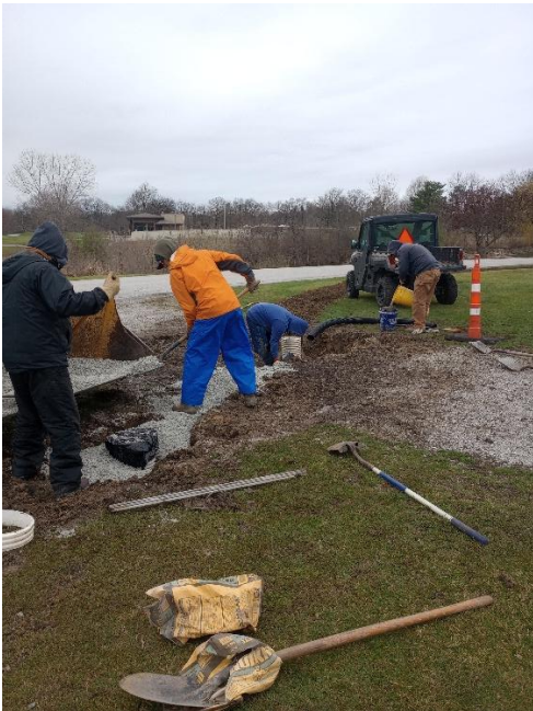
New tile and catch basins at driving range building.
