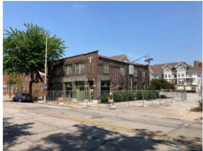
Building at 111 19 th Street, legal work ongoing.
