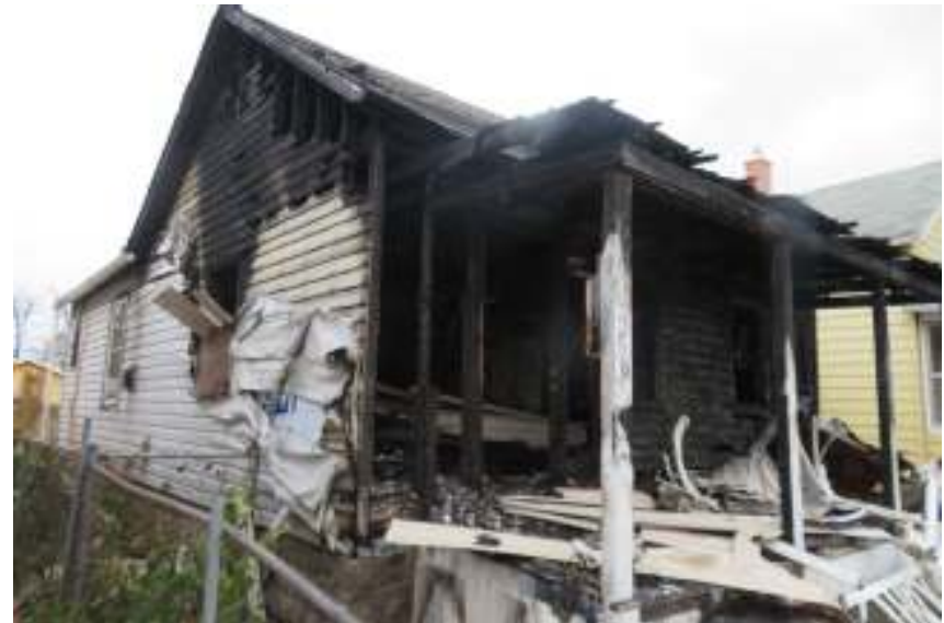
House at 2507 6 th Avenue, demolished in 2022.
