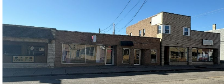
Three vacant spaces along 14 th Avenue, 3822-3830 14 th Avenue
