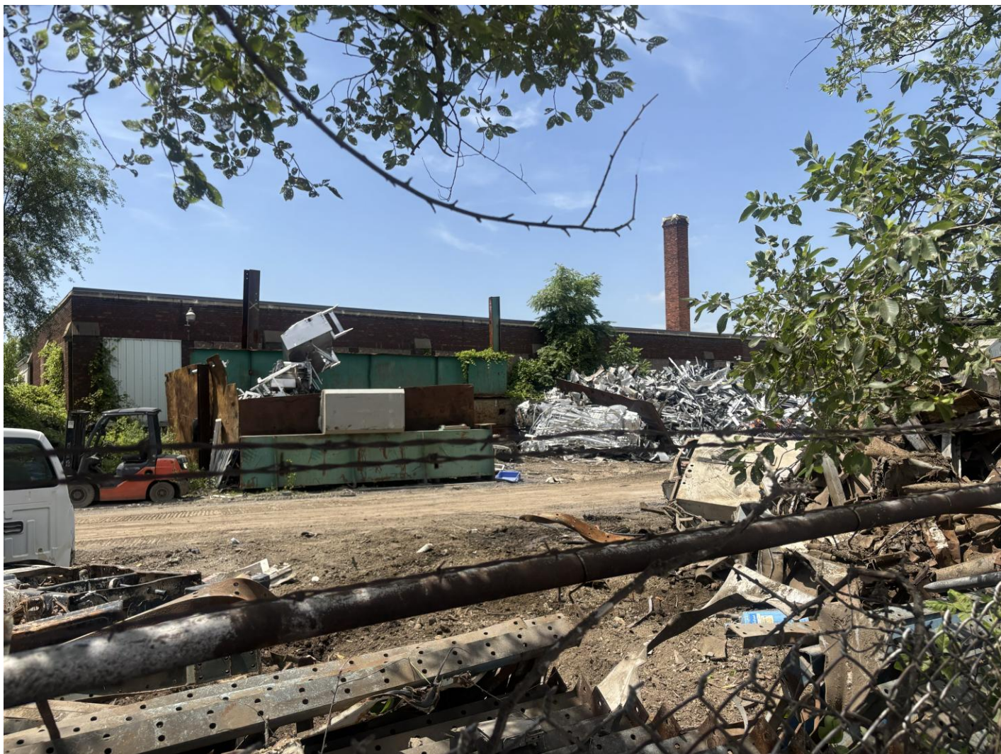
Figure 2: Photo of 1600 Mill Street from 1st Street.
