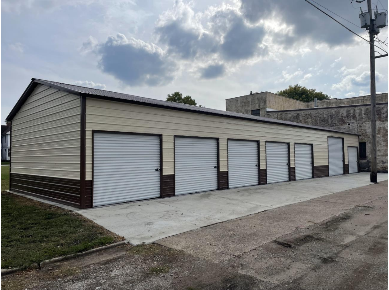
Figure 1: Photo of proposed mini-warehouse building looking southwest.
