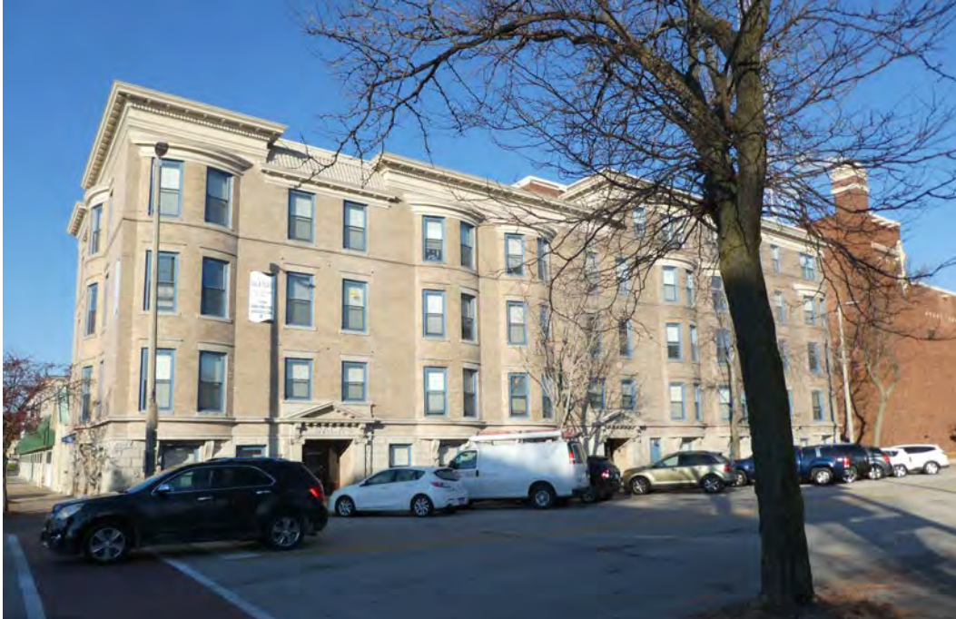
Figure 4. NRHP Resource 3 – 320-330 19 th Street, Sala Apartment Building (NRHP #03000782; City of Rock Island Landmark).
