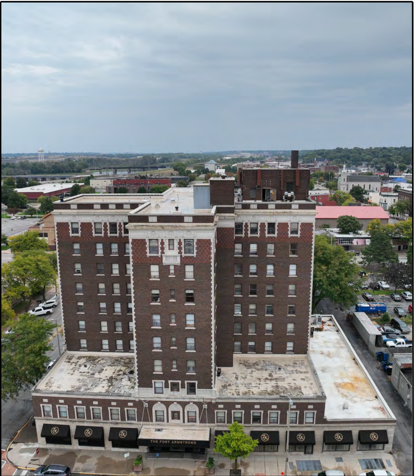
ELEVATION VIEW OF SUBJECT STRUCTURE
