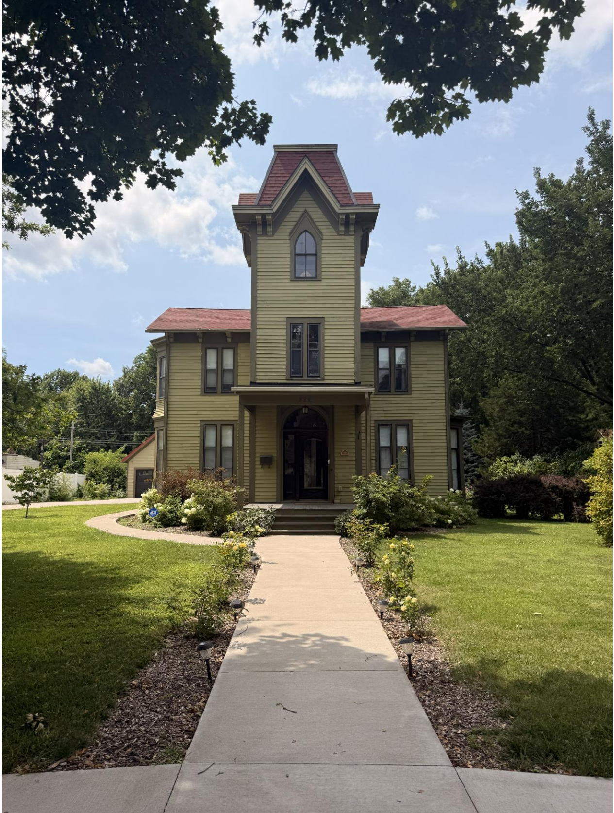
Figure 1: Photo showing front view of the property from along 20 th Street
