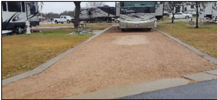
Crushed granite with a concrete edge (acceptable)
