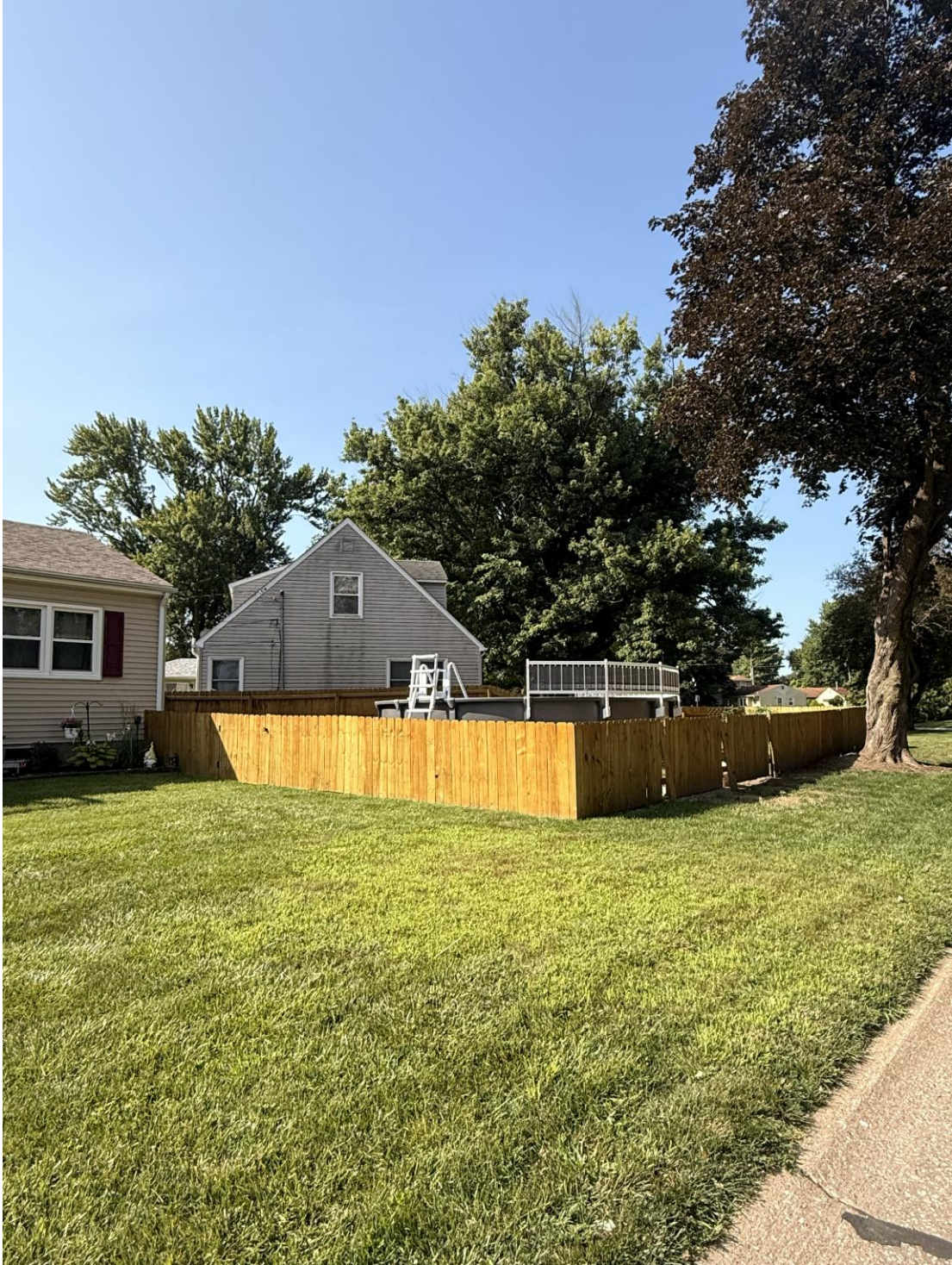
Figure 5. Close-up view of the existing pool located at the subject property.
