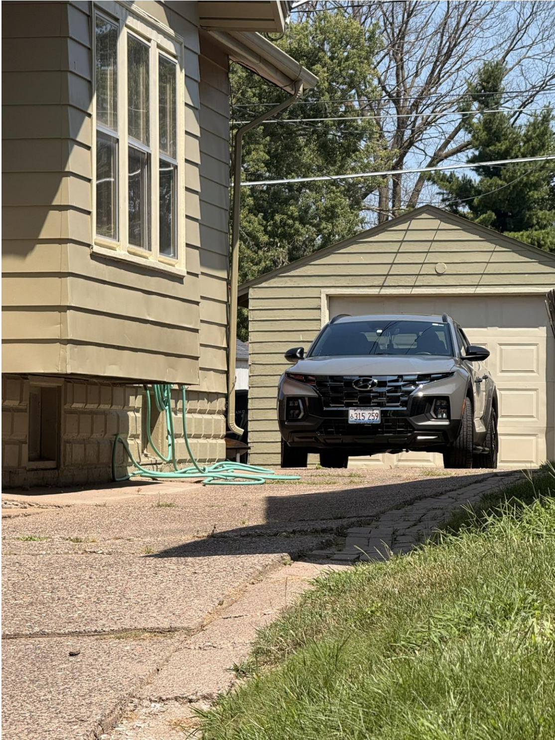
Figure 3. View of the existing garage proposed for replacement.
