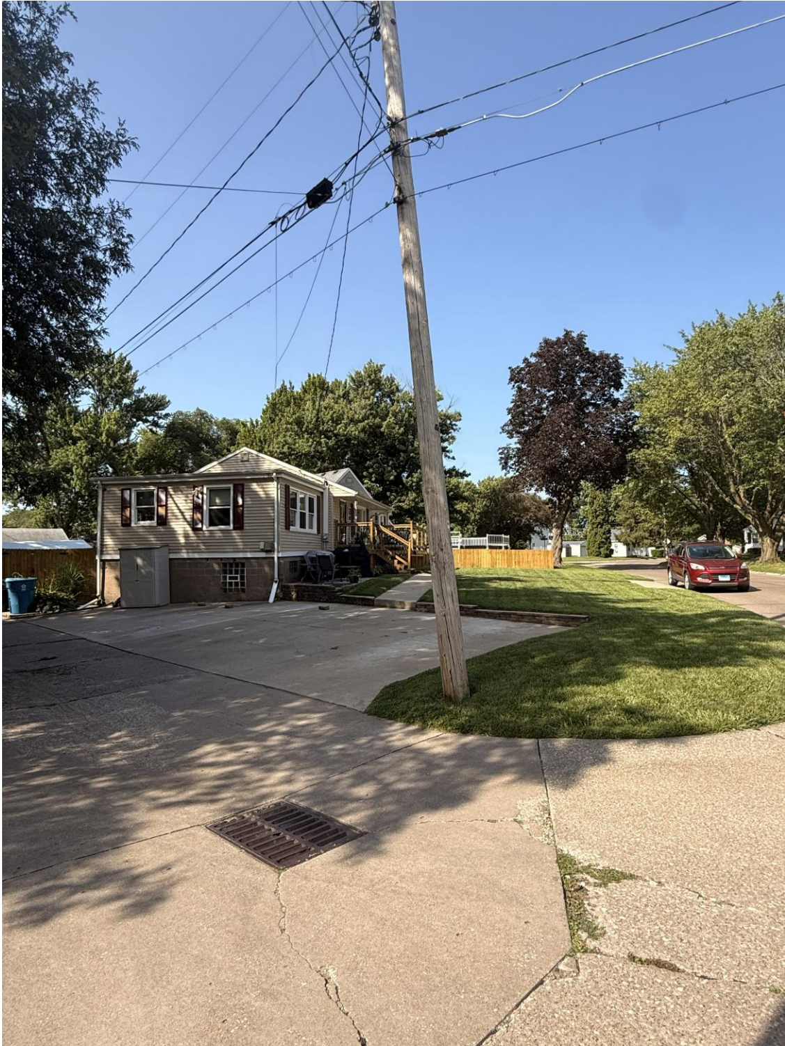
Figure 4. View of the subject property, including the house and pool, as seen from the alley.
