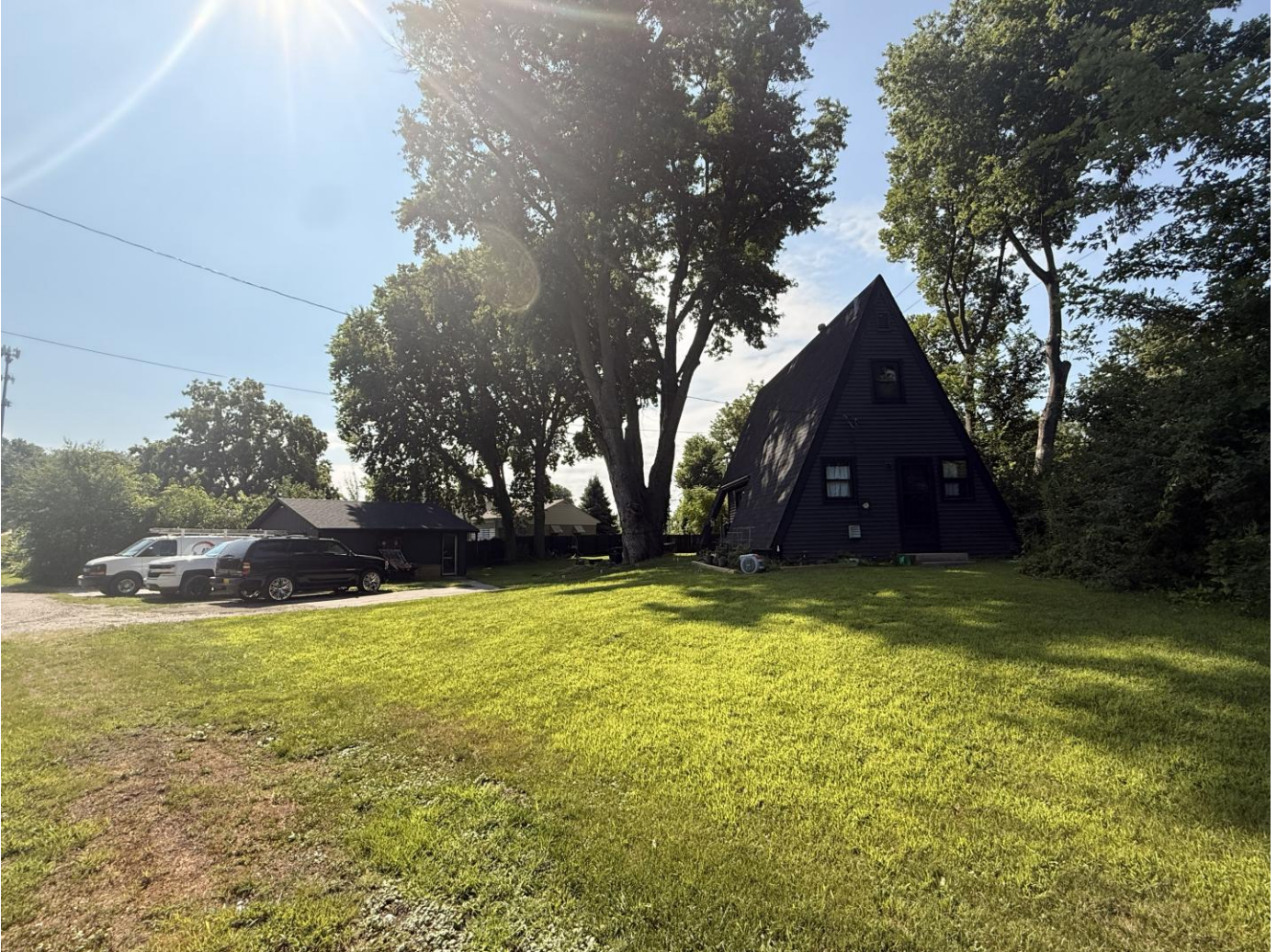
Figure 1. Front view of the property, including the house and garage.
