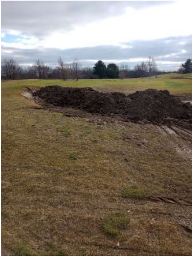
Left side number one green bunker being filled in.
