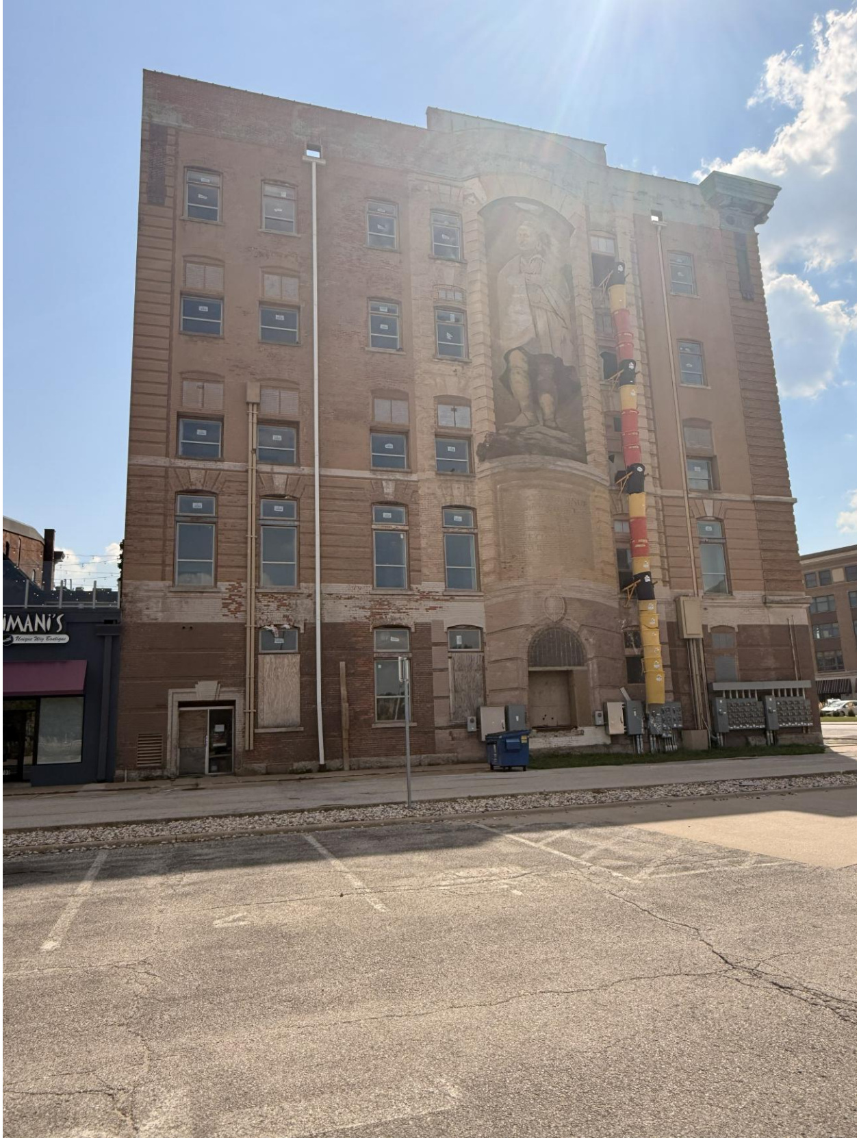
Figure 4: Photo showing the north side (back) of the subject property
