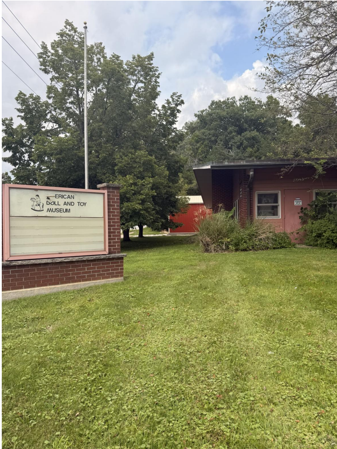
Figure 3: Photo showing how far the accessory structure extends past the main building from along 31 st Avenue
