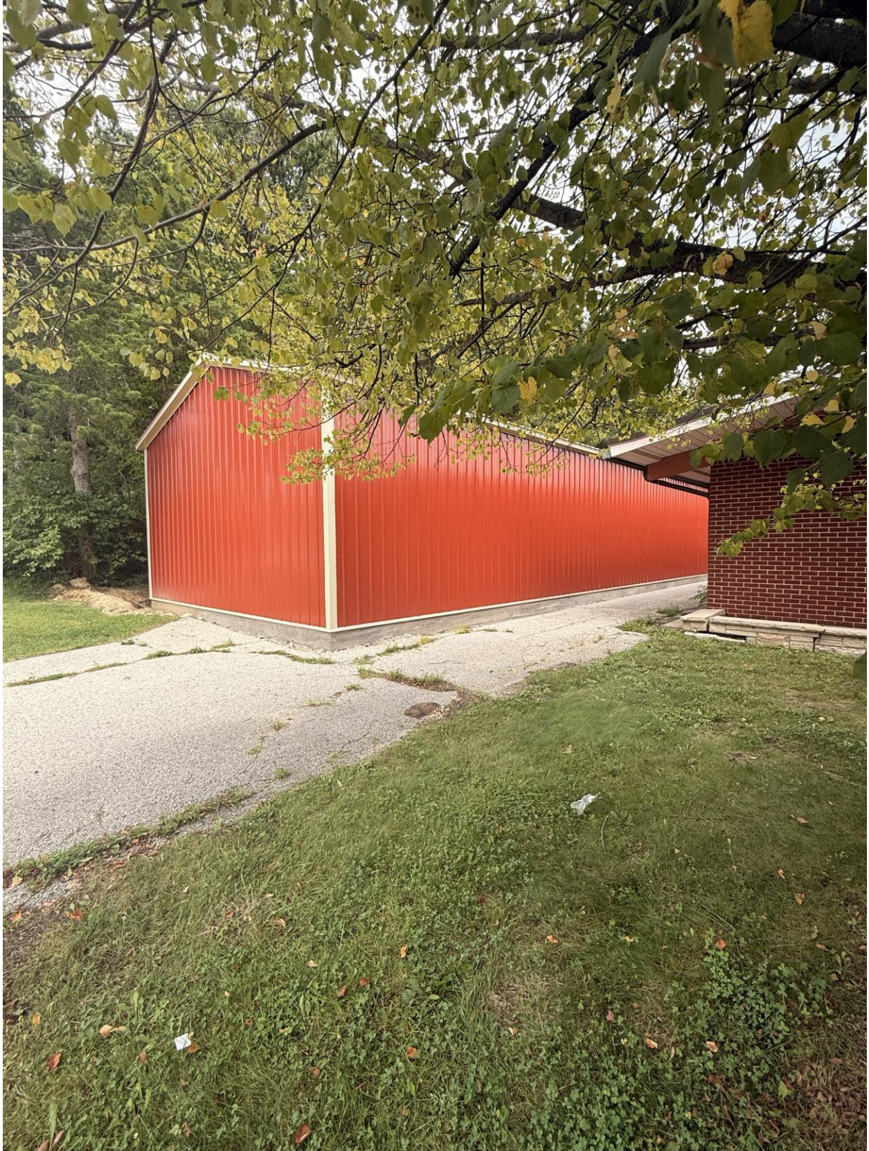
Figure 5: Photo providing a closer look at the structure on the property
