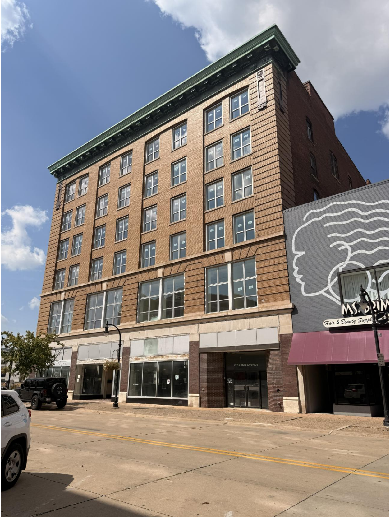
Figure 1: Photo showing the Best Building from along 2 nd Avenue on its southeast end
