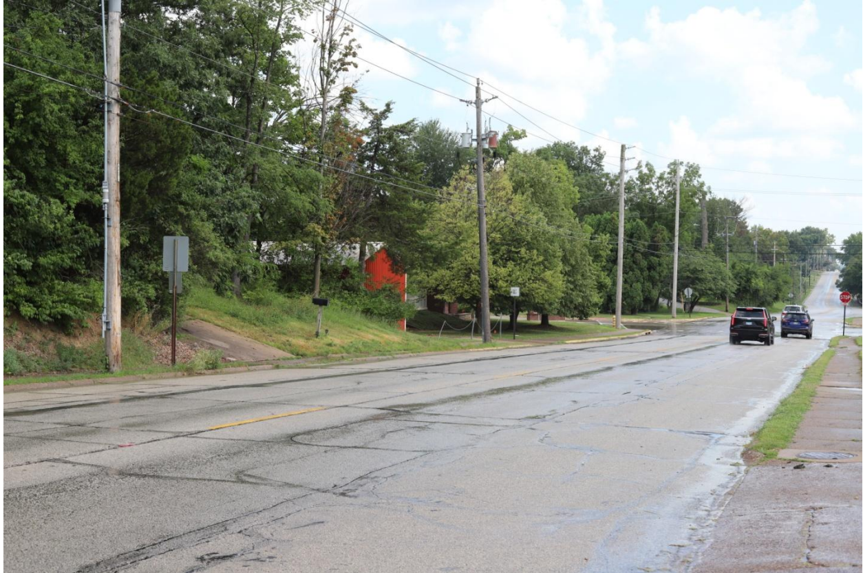
Figure 6: Photo showing the structure from the north perspective along 30th Street
