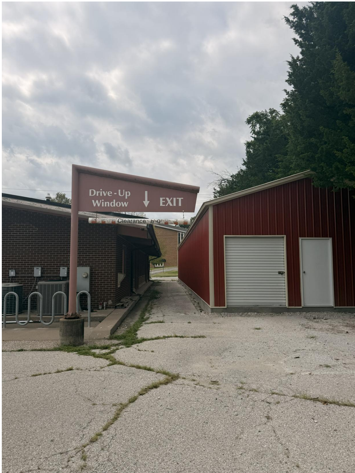
Figure 1: Photo showing the distance between the accessory structure and main building
