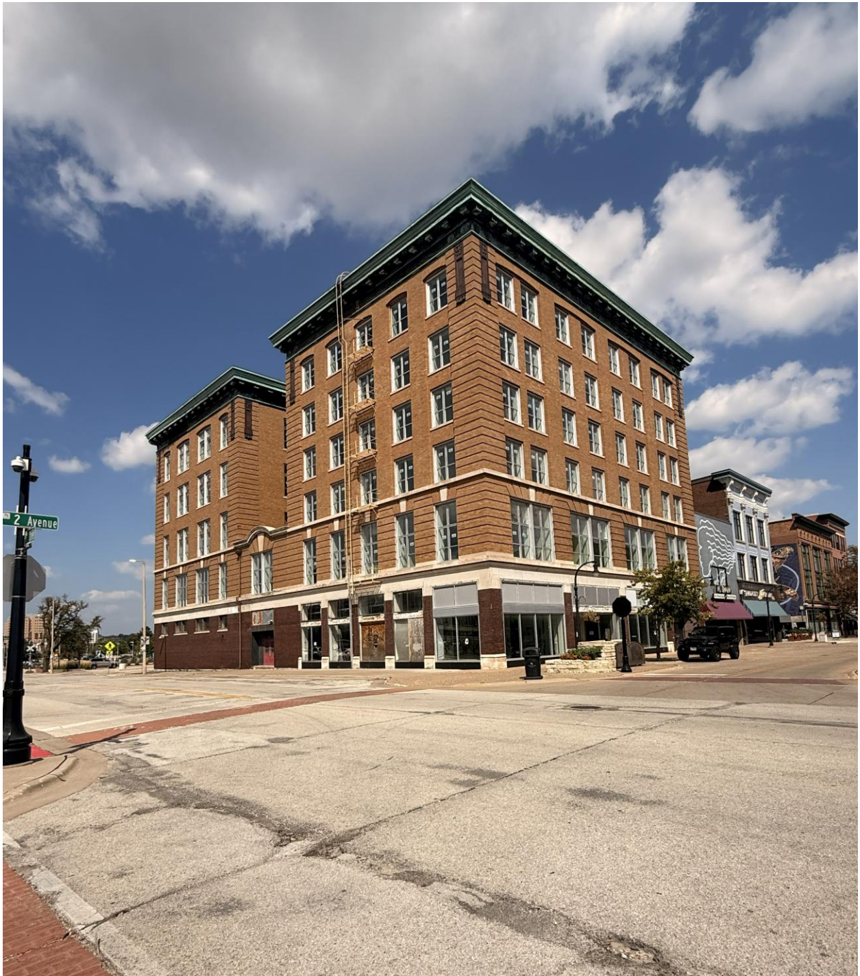
Figure 2: Photo showing the Best Building from the corner of 2 nd Avenue and 17 th Street
