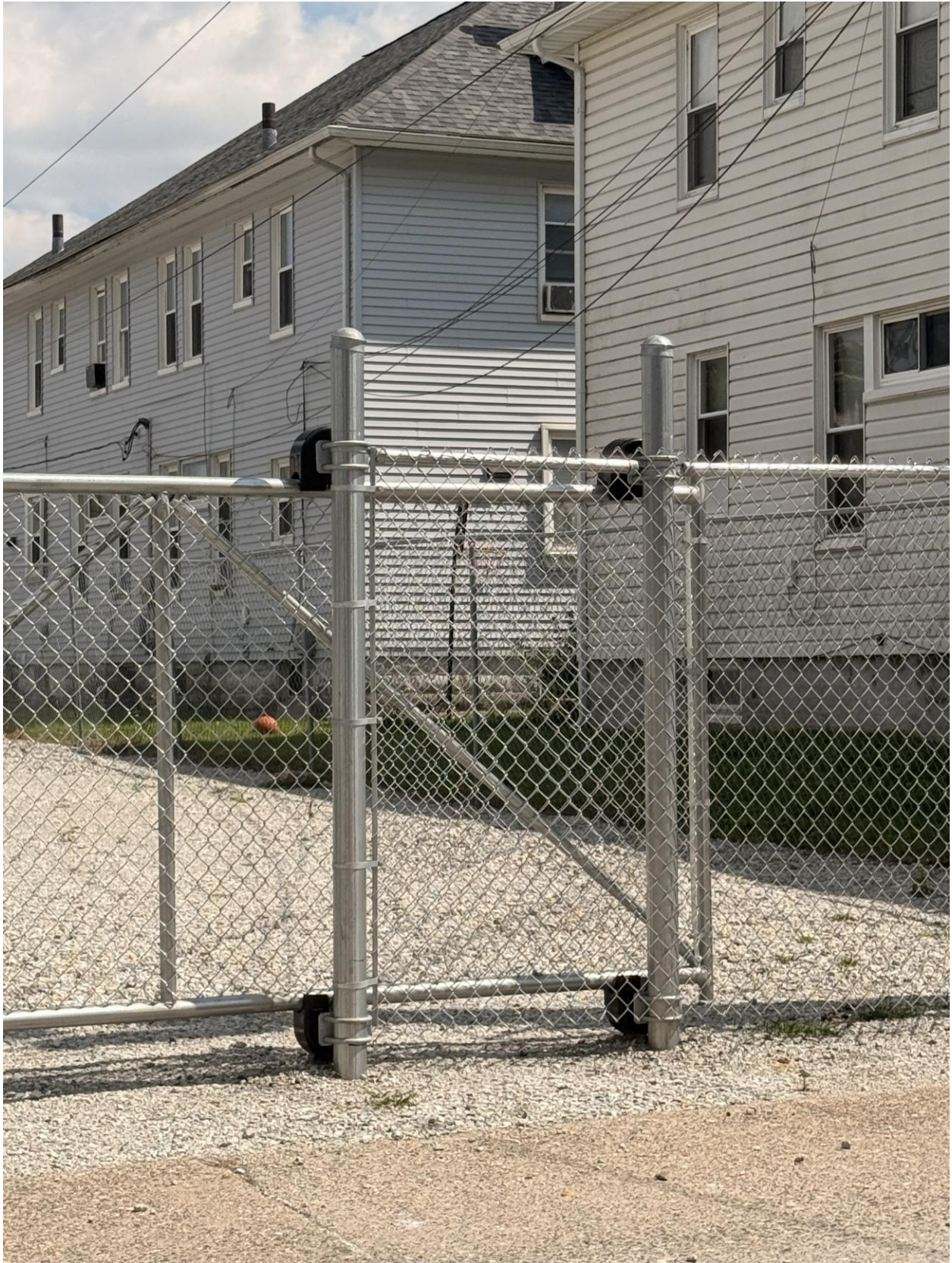
Figure 3: Photo showing the gate on the fence
