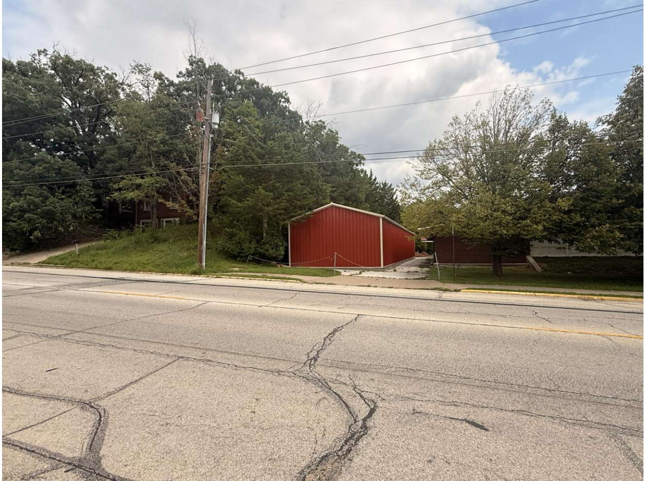
Figure 2: Photo showing structure from across 30 th Street
