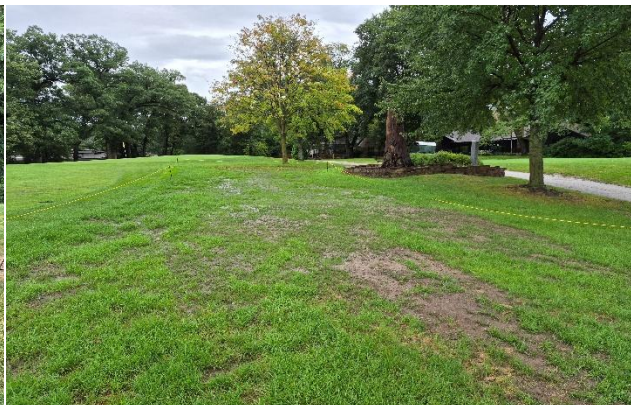
#4 rough after being backfilled and seeded
