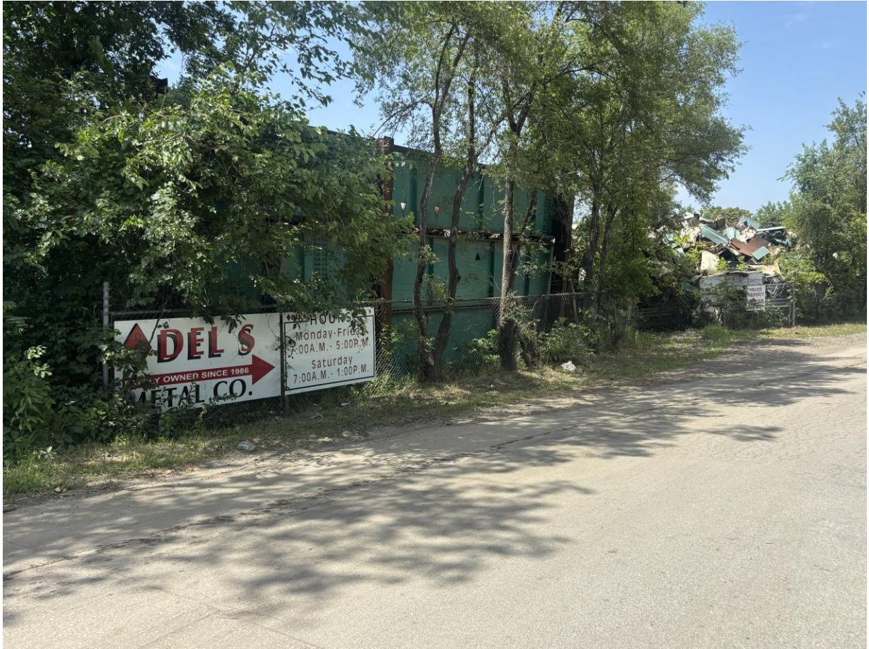
Figure 1: Photo of 1600 Mill Street looking northwest from 18 th Avenue & 1 st Street.
