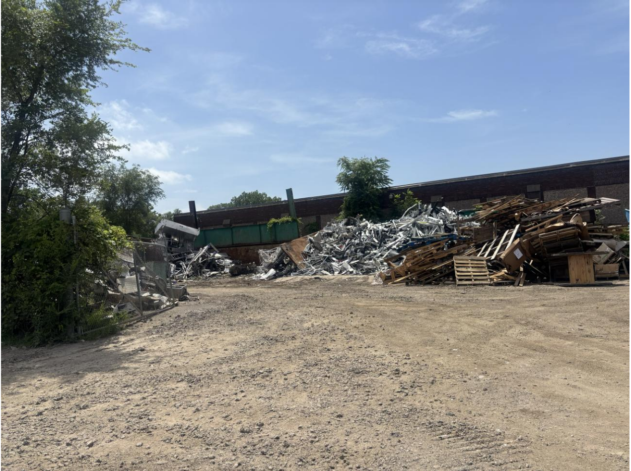
Figure 4: Photo of 1600 Mill Street showing access point from 1st Street.
