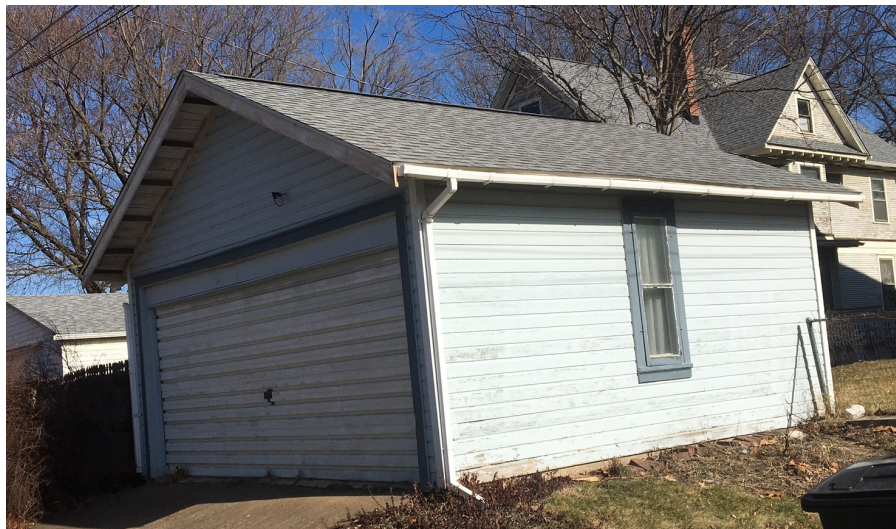
Fig 14. SW View Garage
