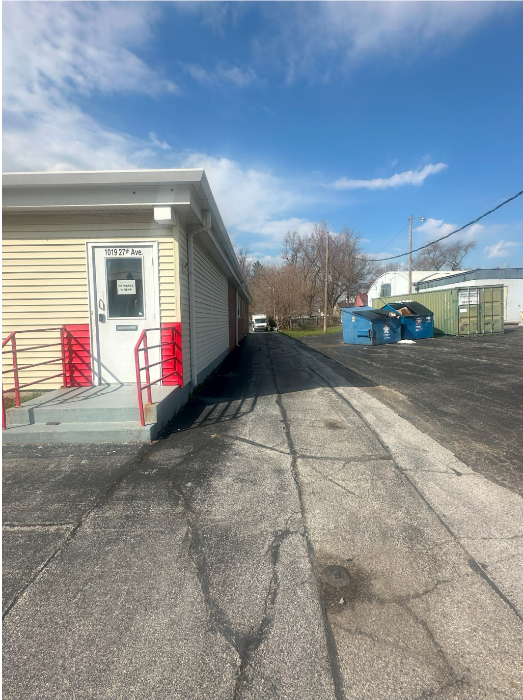
Figure 2: View of access along the east side of the building
