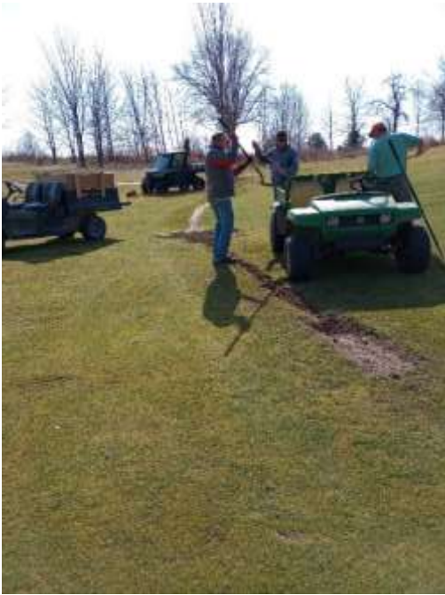
Staff installing new drain tile in the valley of eighteen.
