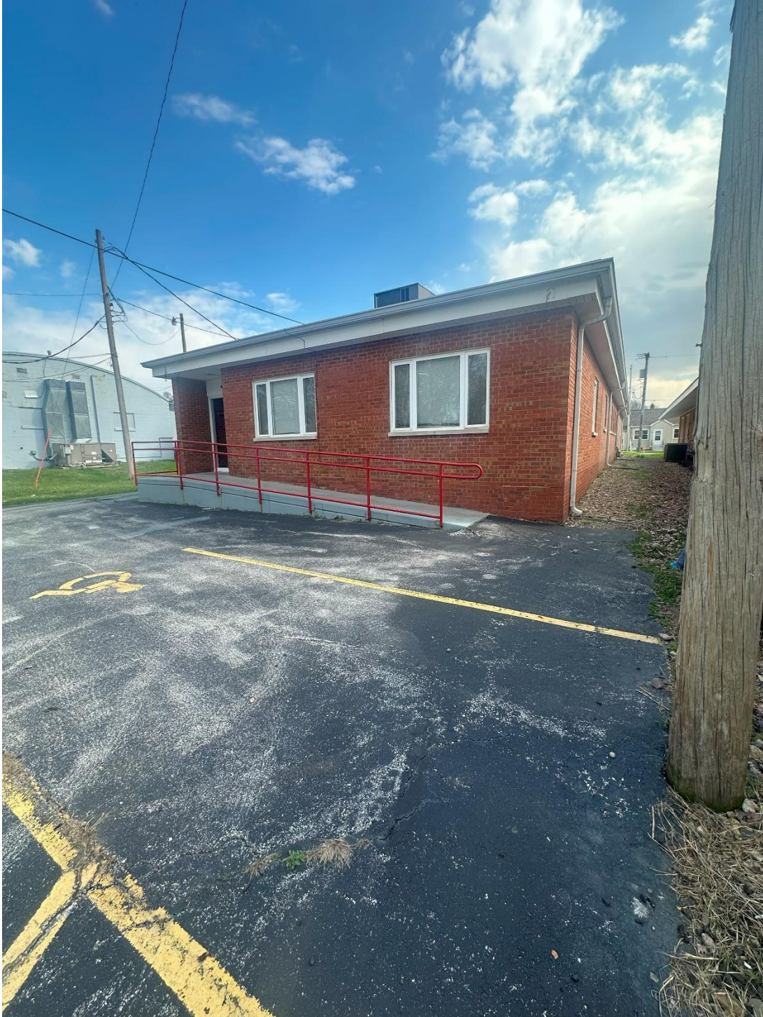
Figure 4: View of the ADA-accessible parking, ramp and east side access
