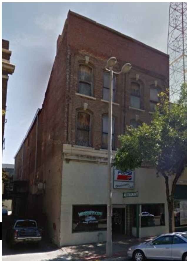
Fig. 3. Dart Warehouse, 2011 Google Maps
