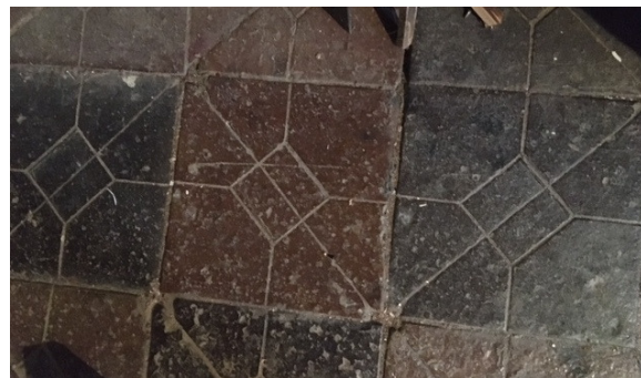
Fig. 7 Basement Floor Pavers
