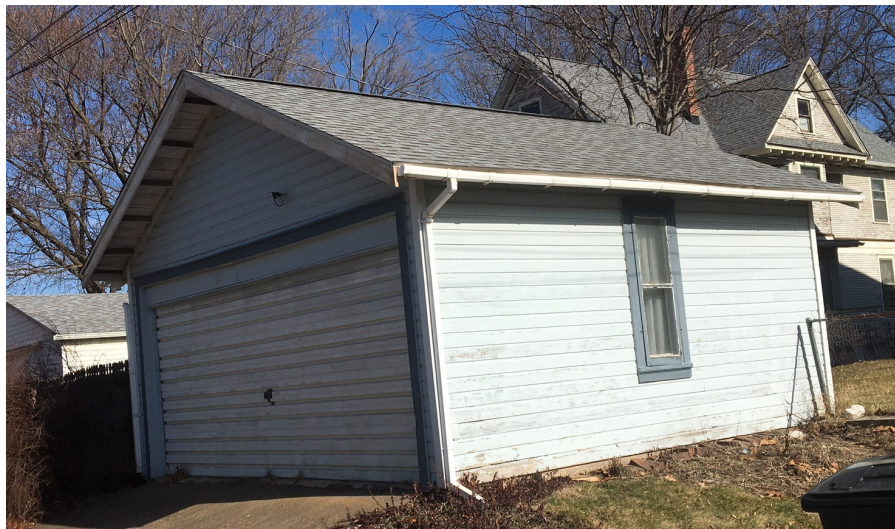
Fig 14. SW View Garage
