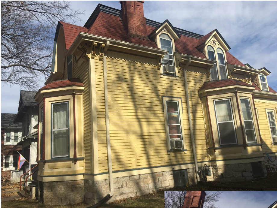
Fig 8. SE Corner View
