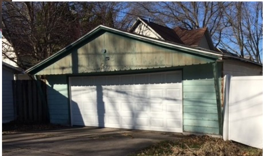
Fig. 13. 1979 Garage NE View
