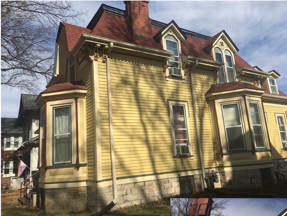
Fig 8. SE Corner View
