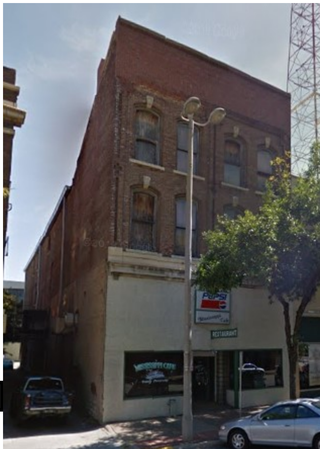
Fig. 3. Dart Warehouse, 2011 Google Maps
