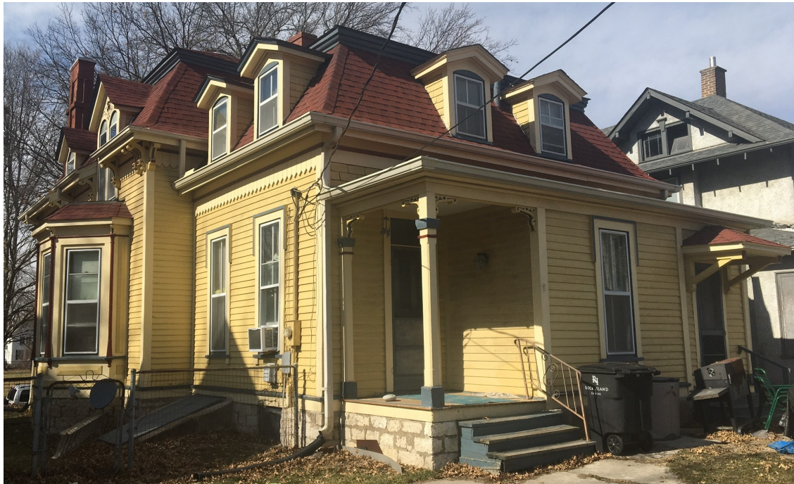
Fig 11. SE Corner View
