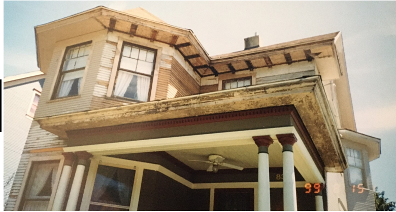
Fig. 4. Great Unveiling, West Side Showing Missing Modillions
