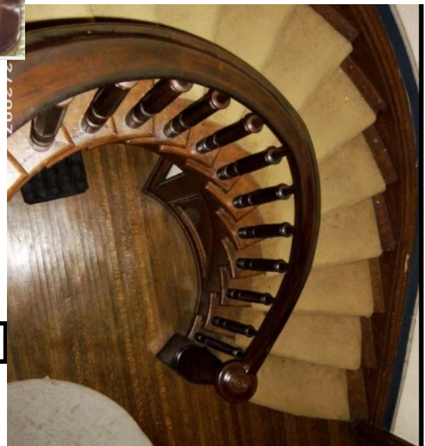
Fig 14. Staircase from Above
