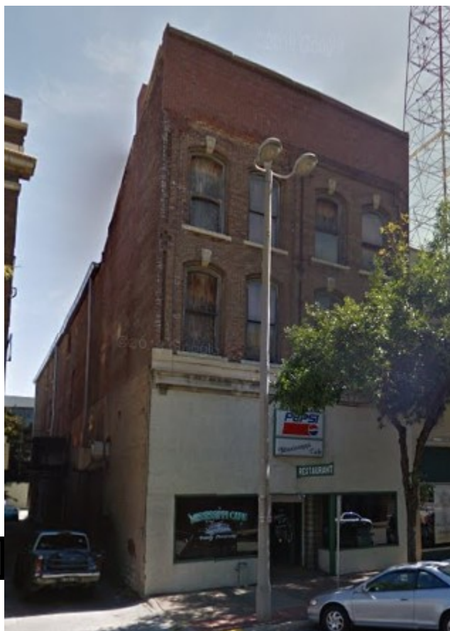
Fig. 3. Dart Warehouse, 2011 Google Maps
