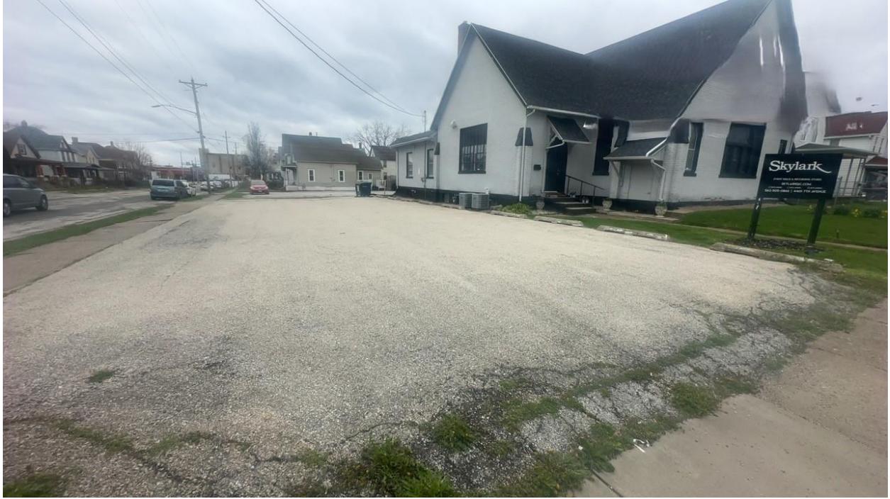
Figure 1: Photo showing paved parking area for the business
