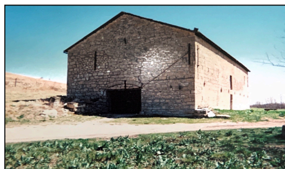
Figure 4. Post Rock Structure. Source: Kansas Historical Society
