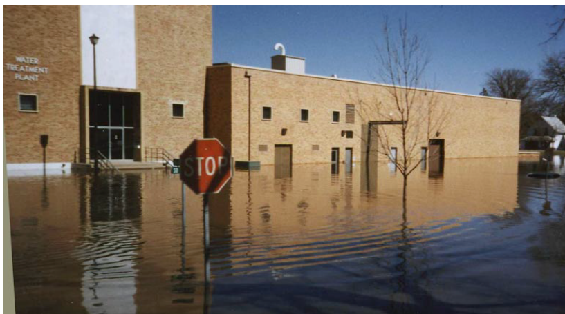
Figure 5. Grand Forks Water Treatment Plant, 1997. Source: FEMA.
