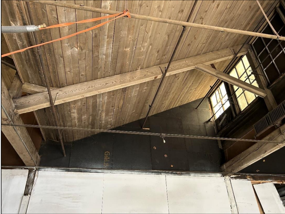
Photo 25 – Sawtooth Roof Framing Members
