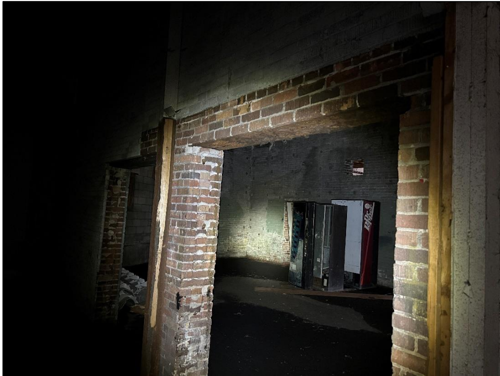
Photo 36 – Interior Wall w/ Opening and Steel Lintel
