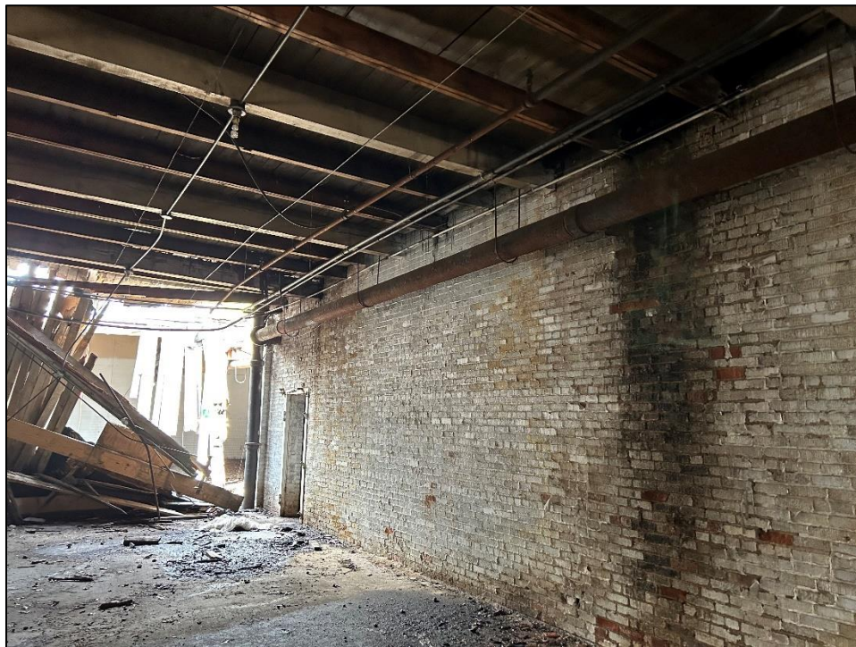
Photo 42 – Interior Brick Wall Between Zones 2 & 3
