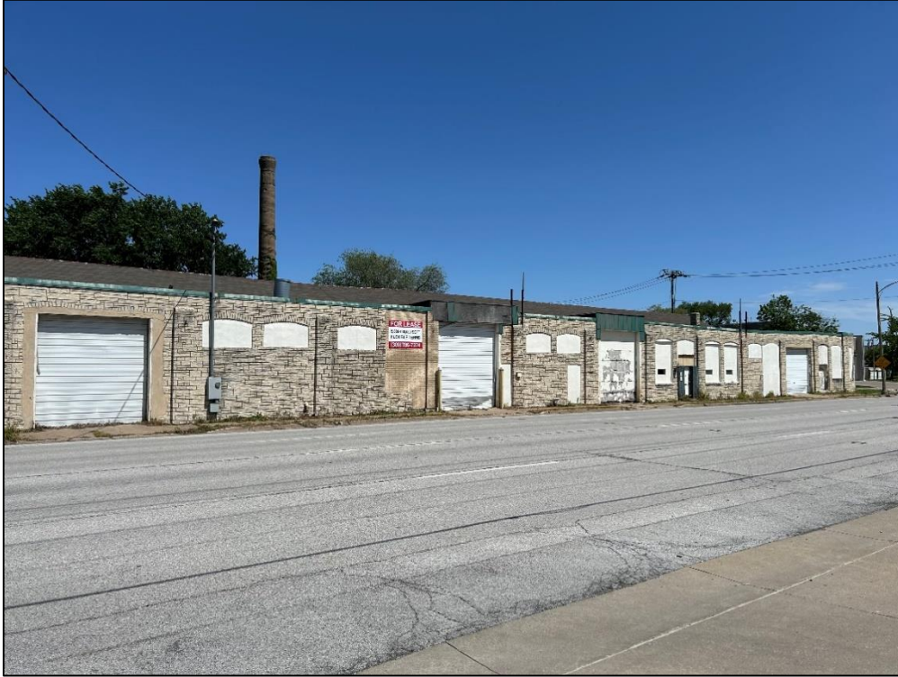
Photo 1 – Overall South Face of Structure
