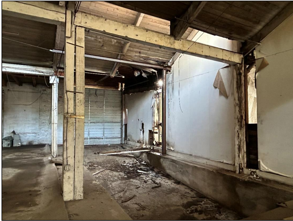
Photo 44 – Steel Reinforcing of Timber Beam
