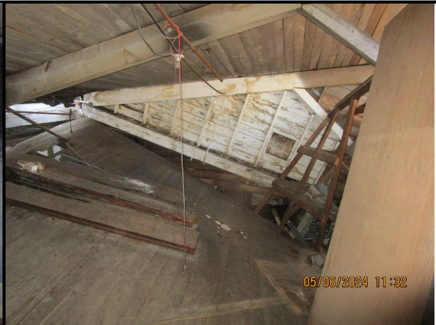
Photo 16: View of collapsed roof in dock area. Collapsed sections of the roof were observed throughout the building.
