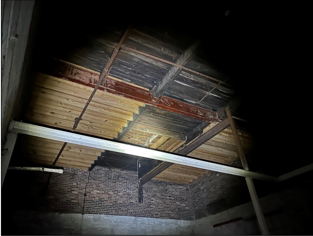
Photo 33 – Steel Roof Beam with Repaired Infill Joists
