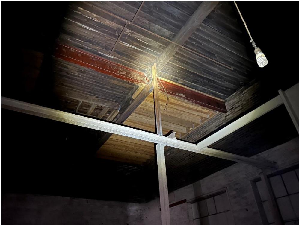
Photo 34 – Steel Roof Beam with Repaired Infill Joists
