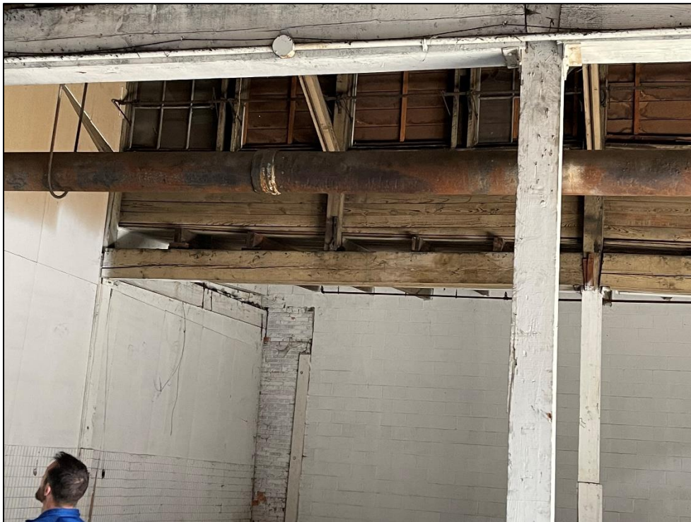
Photo 56 – Checking of Beam Members, Separation of Joists and Beam
