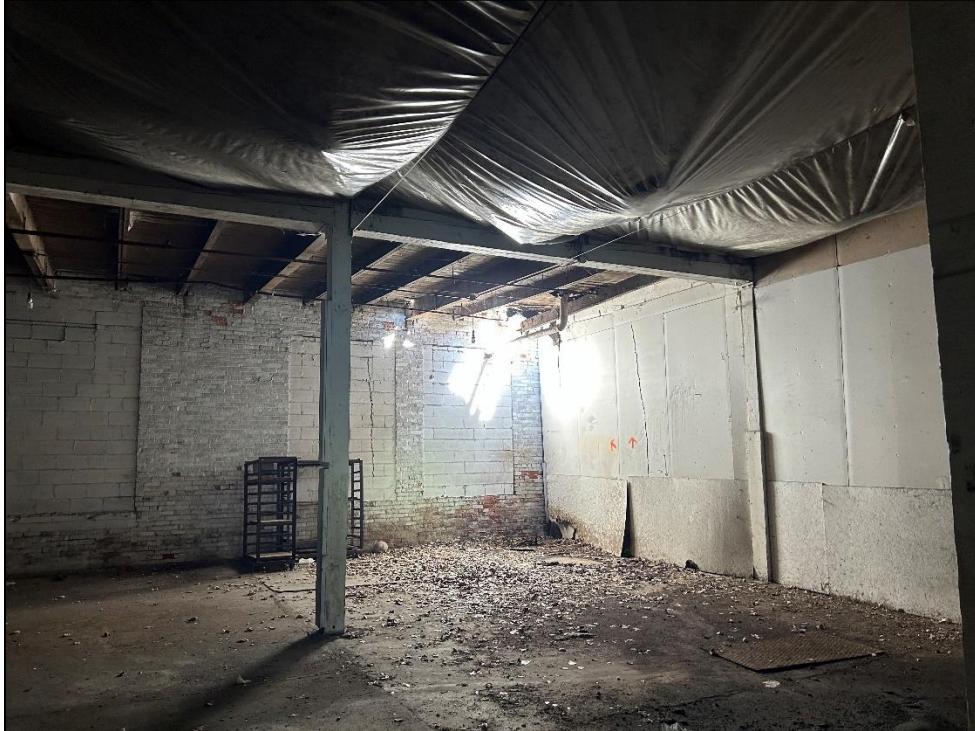
Photo 67 – Collection of Weight in Plastic Ceilings
