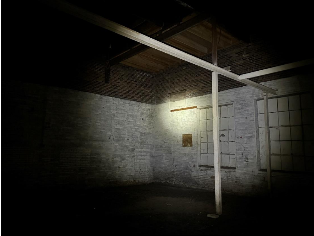
Photo 31 – Steel Beam Framing in Zone 2
