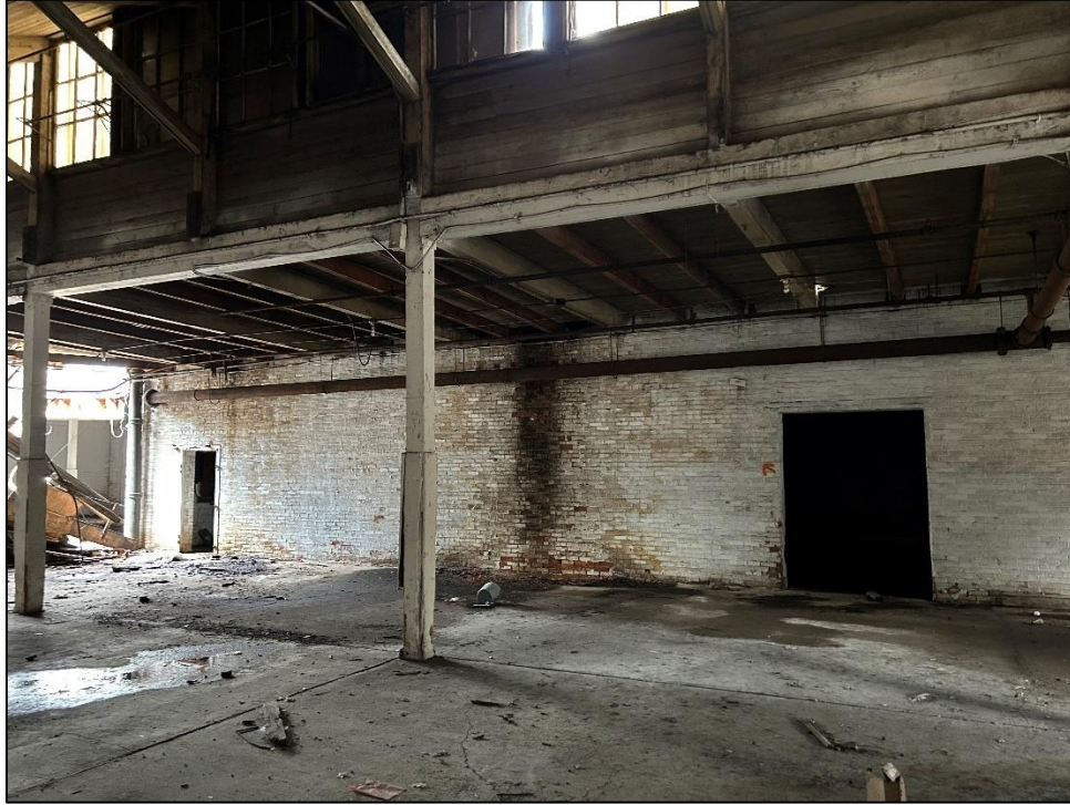
Photo 39 – Flat Roof Members Outside Zone 2
