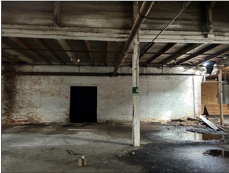
Photo 38 – Flat Roof Members Outside Zone 2
