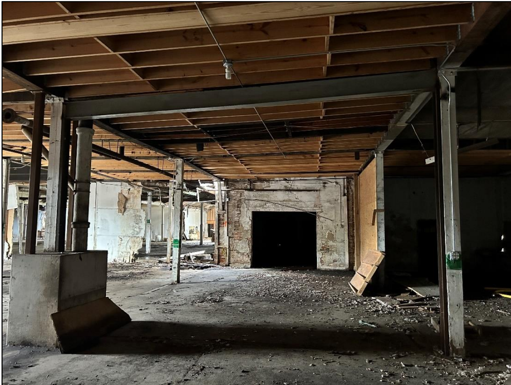
Photo 16 – Steel Beam Reinforcing in Zone 1 North End
