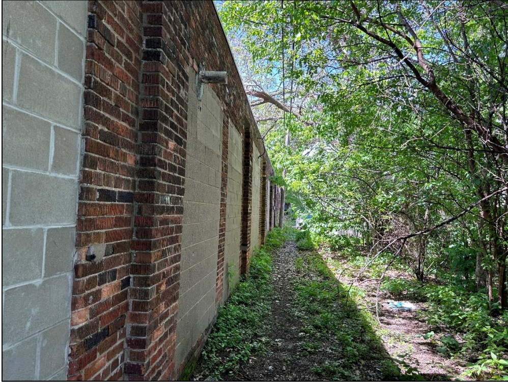
Photo 3 – North Face Exterior Wall
