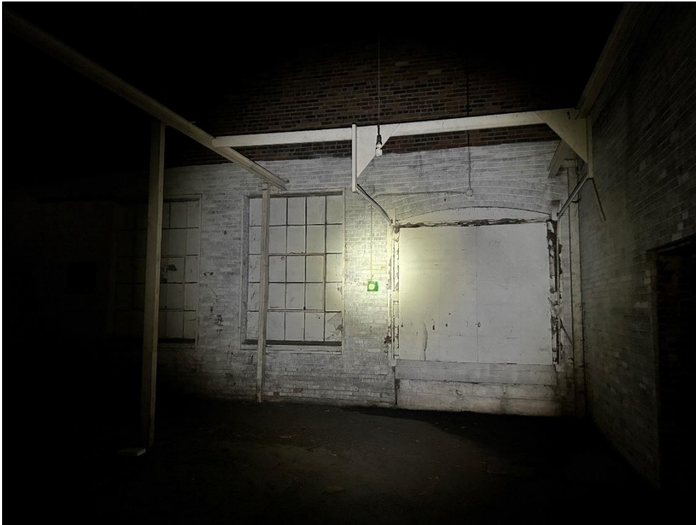
Photo 32 – Steel Beam Framing in Zone 2
