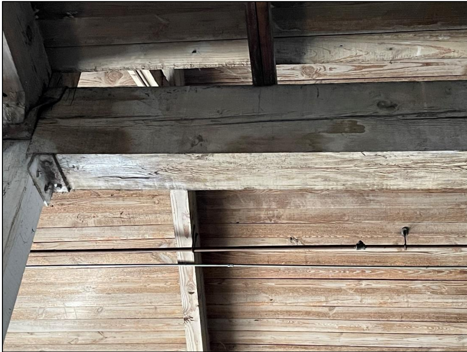
Photo 60 – Checking of Timber Beam Members
