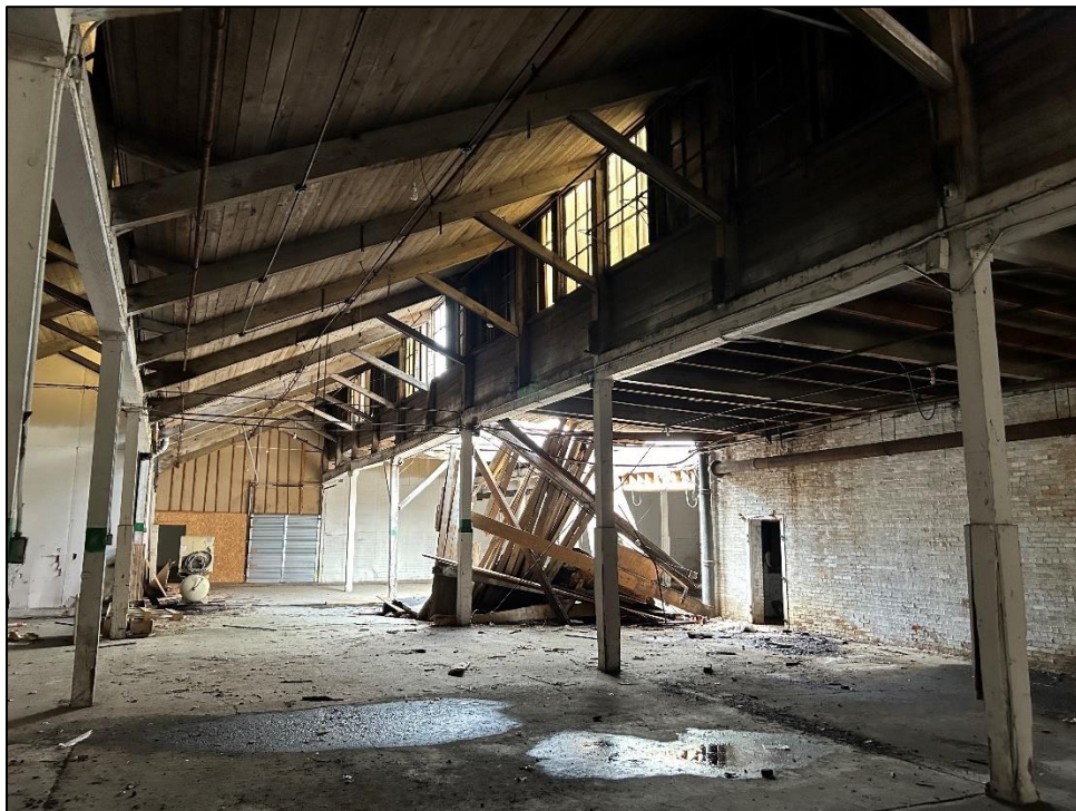
Photo 40 – General View of Zone 3
