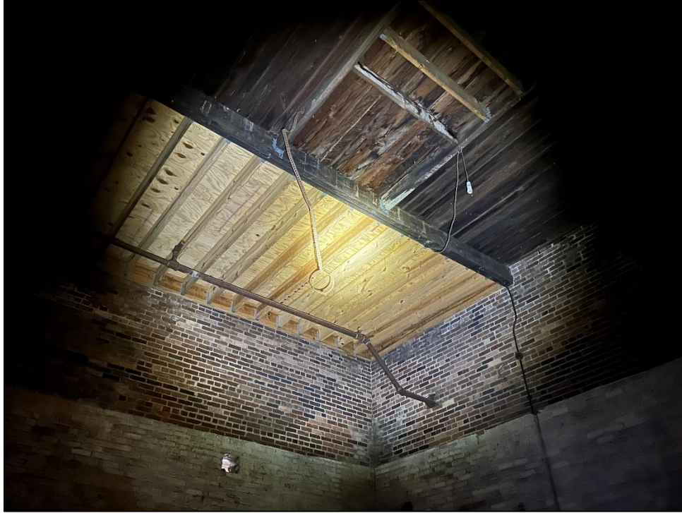
Photo 37 – Repair of Roof Infill
