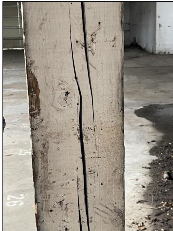
Photo 28 – Checking of Timber Columns
