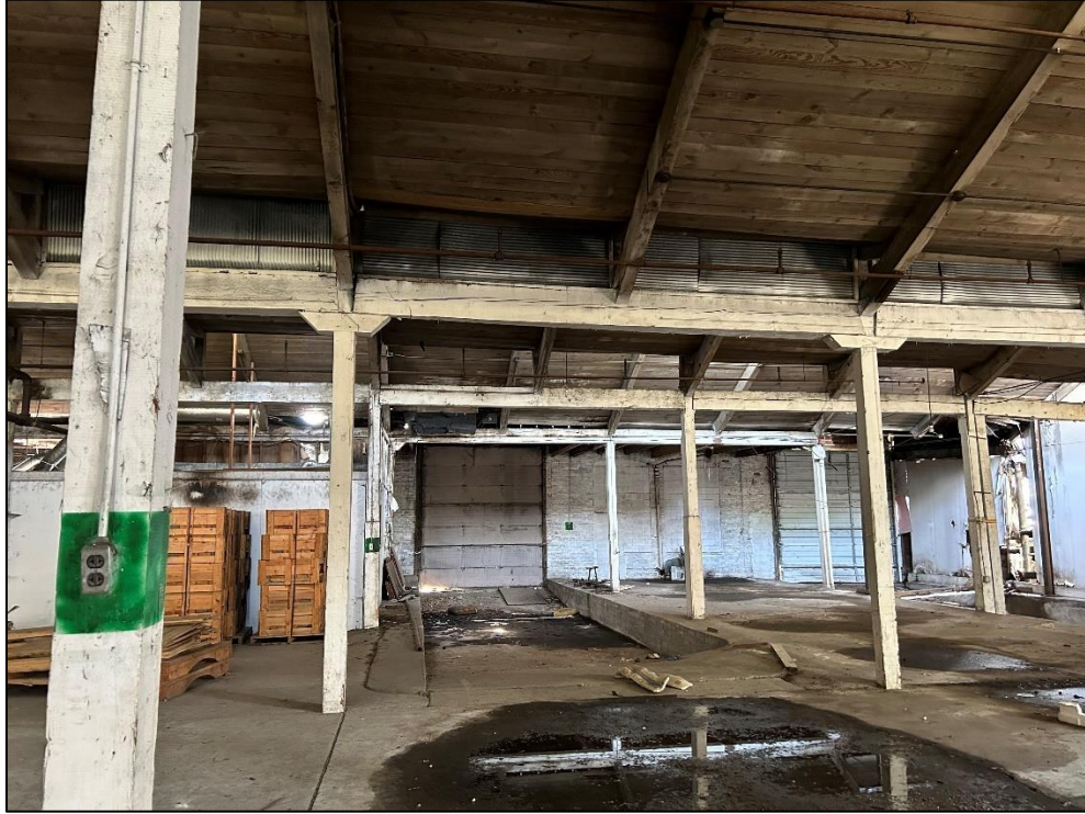
Photo 43 – Loading Bays in Zone 3
