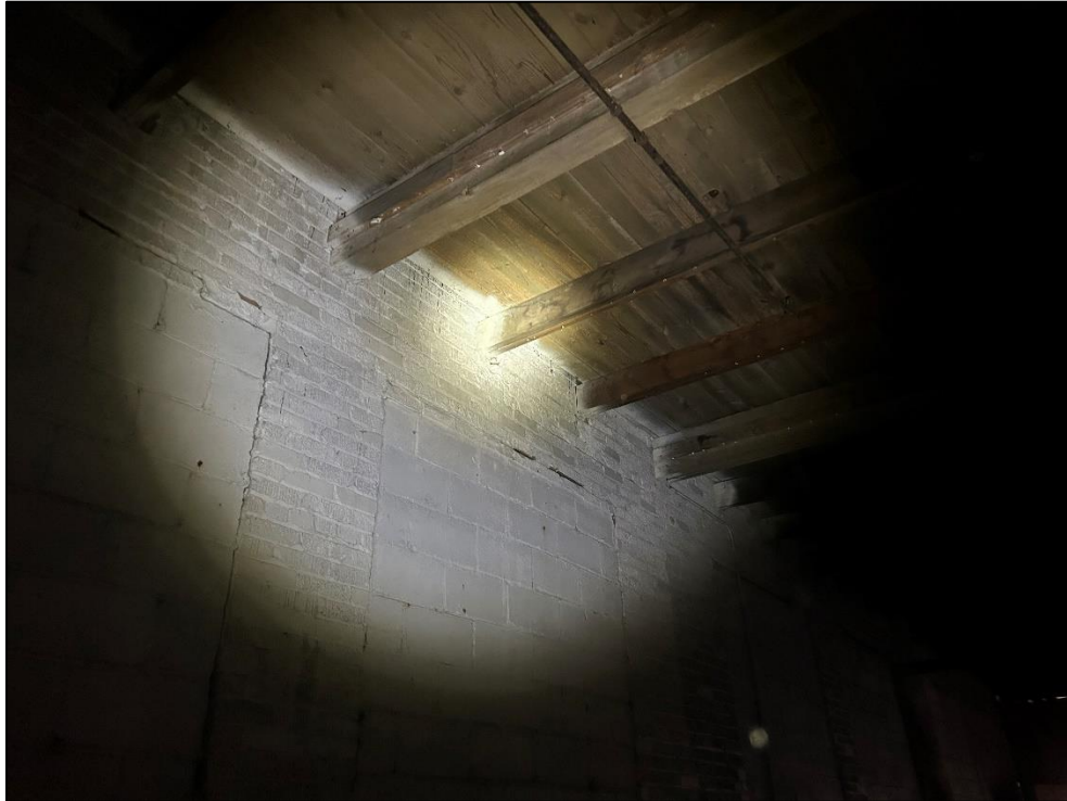
Photo 73 – Joist Beam Pockets in Exterior Wall
