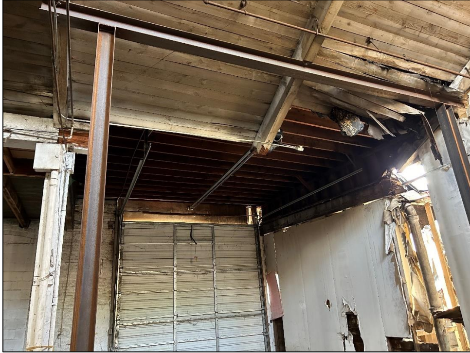
Photo 45 – Steel Beam and Column Framing Replacing Broken Timber Beam
