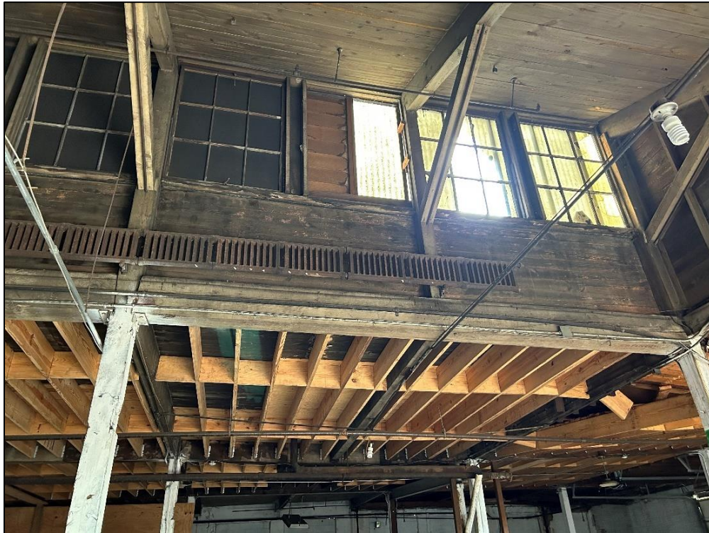
Photo 24 – Replaced Roofing Infill Members
