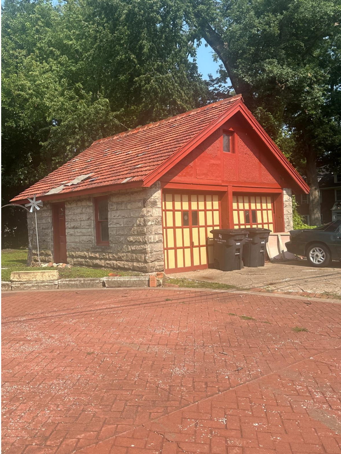
Figure 1: Photo showing overall view of the garage from along the alleyway
