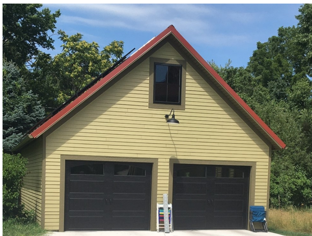
Fig.18. Garage, Front East Side (below)
