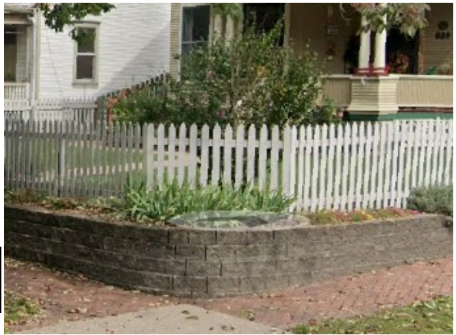
Fig. 10. Retaining Wall, Fence, & Brick Sidewalk 607 W. Edgington
