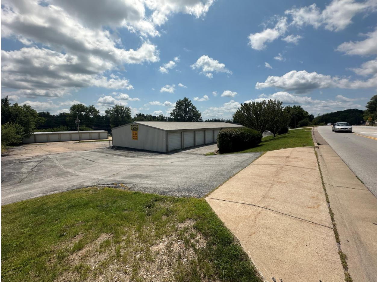
Figure 2: Photo showing the east side of the property from along Blackhawk Road.
