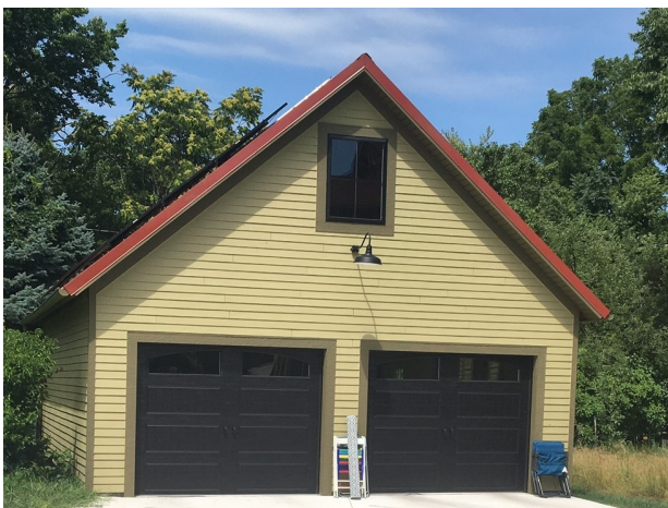
Fig.18. Garage, Front East Side (below)
