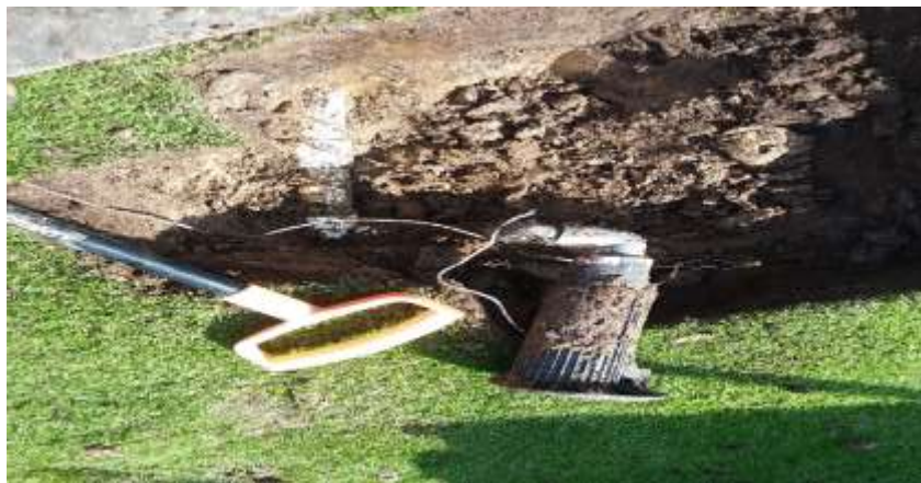
Irrigation head being repaired
