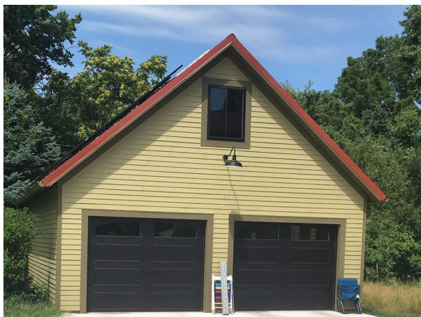
Fig.18. Garage, Front East Side (below)
