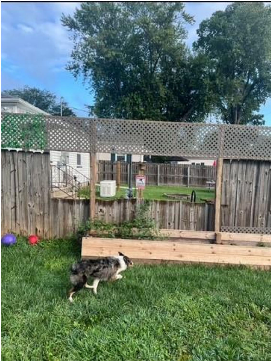
Figure 1: Photo showing section of fence for 8ft install
