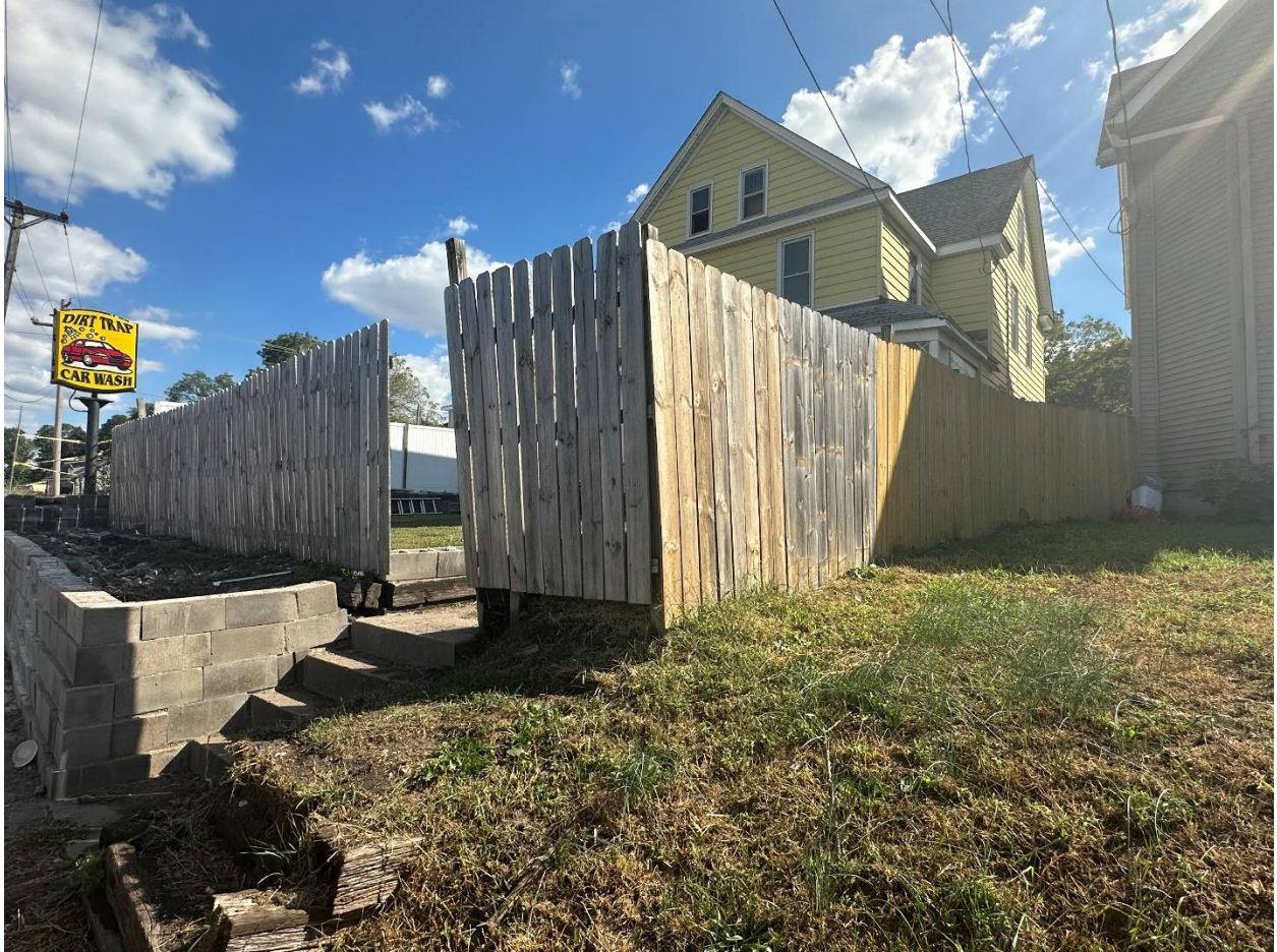
Figure 1: A photo showing the 6-foot fence in the front yard along 5 th Avenue
