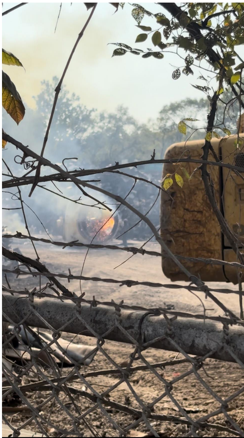
Figure 8: Photo of 1600 Mill Street showing worker cutting metal.
