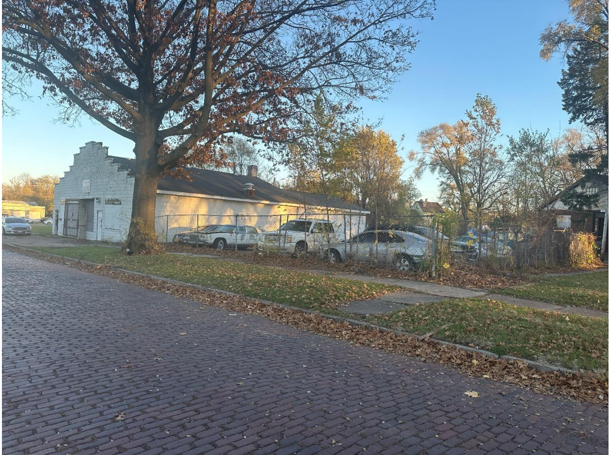
Figure 2: Photo showing properties 1000-1006 8 th Avenue from the corner of 10 th Street and 8 th Avenue
