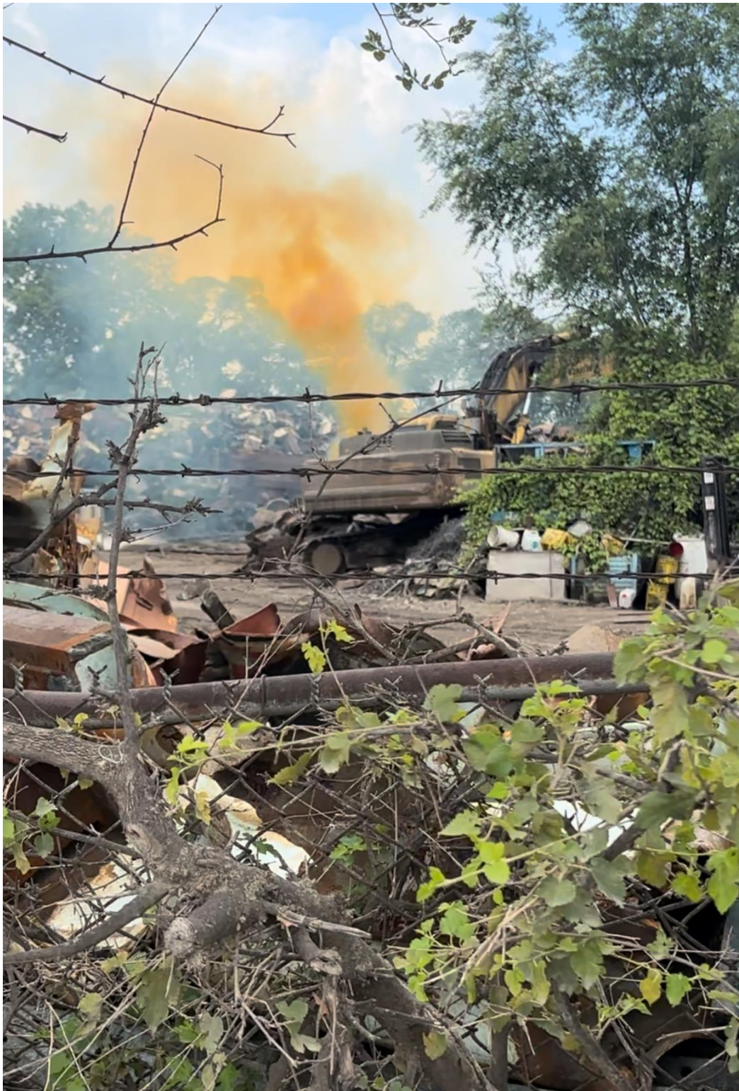
Figure 7: Photo of 1600 Mill Street showing orange smoke from presumed metal cutting.
